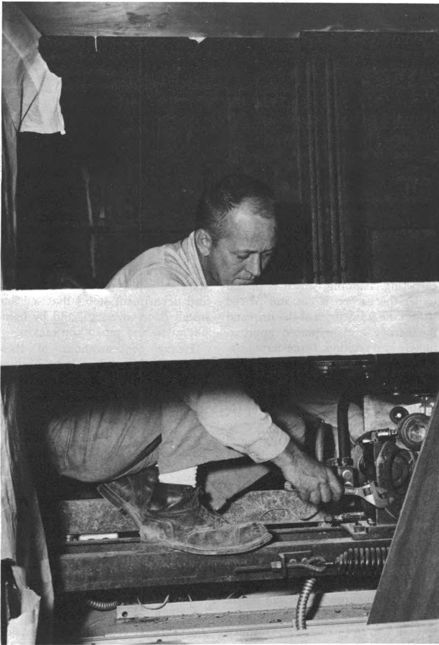
Elevator constructor adjusts mechanism that operates elevator doors.
