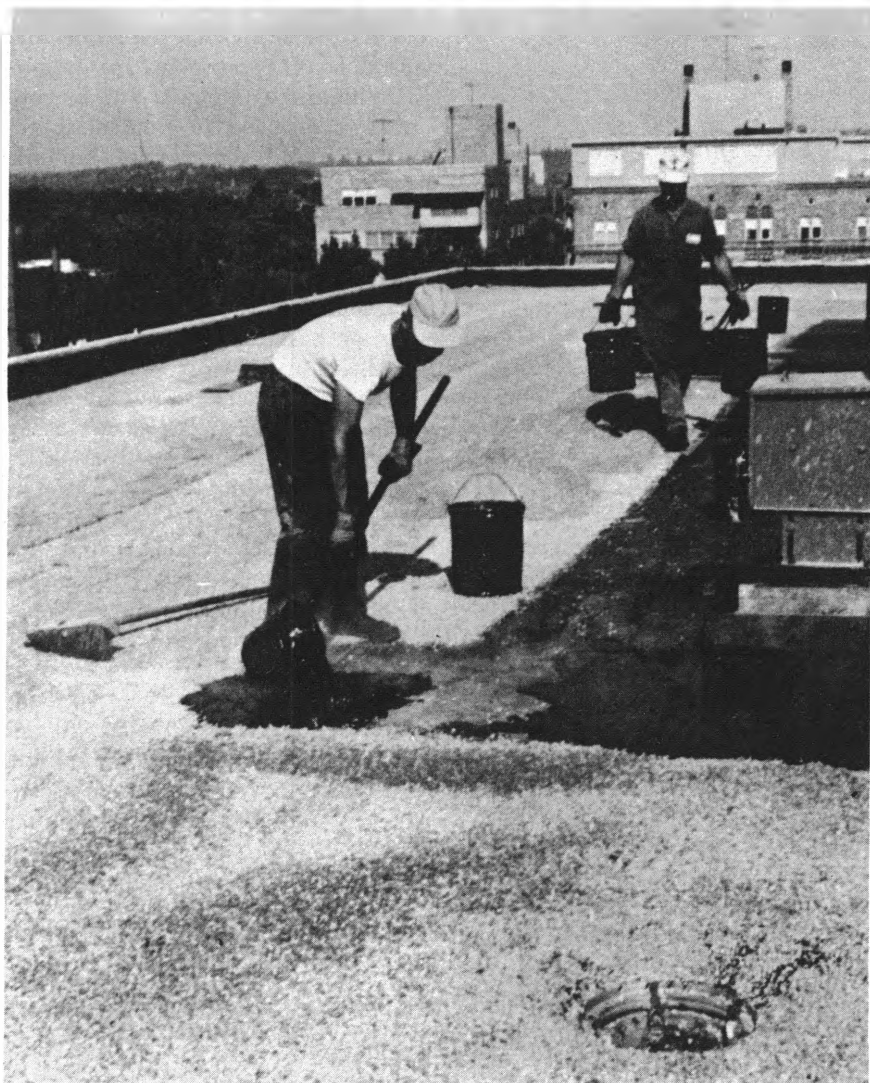
Roofers apply tar prior to spreading gravel.
