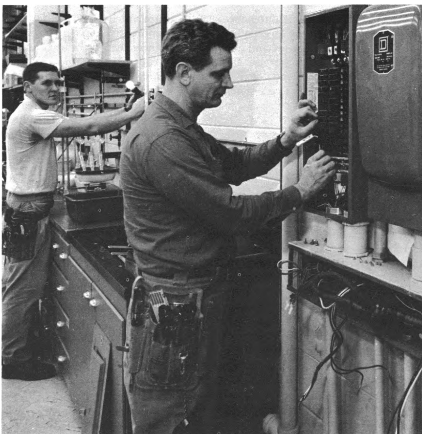
Electricians install new circuits.
