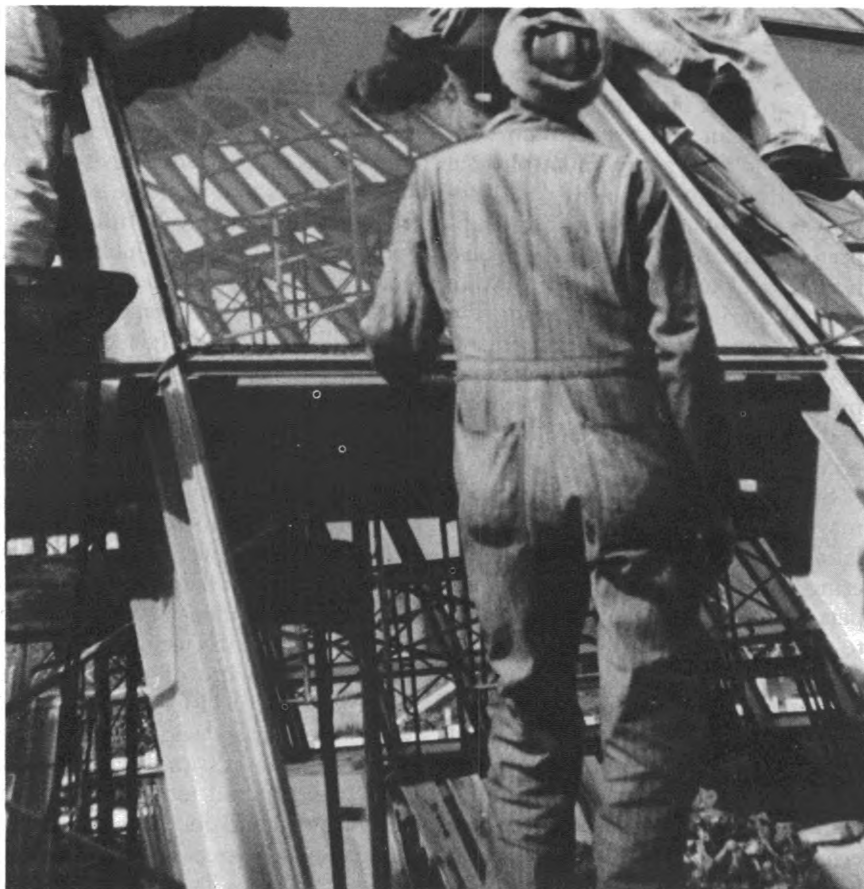
Glaziers position glass panel.
