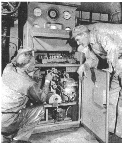
Manufacturer's service representative instructs mechanic in maintenance of refrigeration controls.
