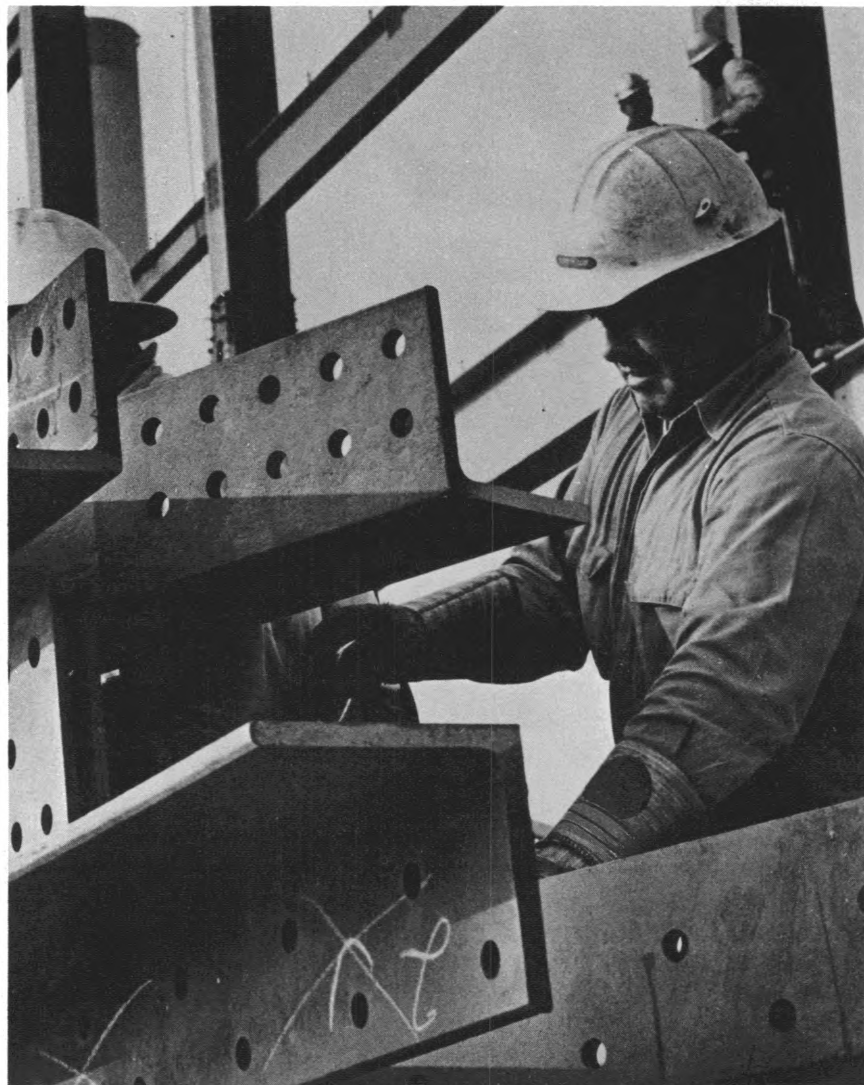
Structural-iron workers wrestle heavy girders into position.
