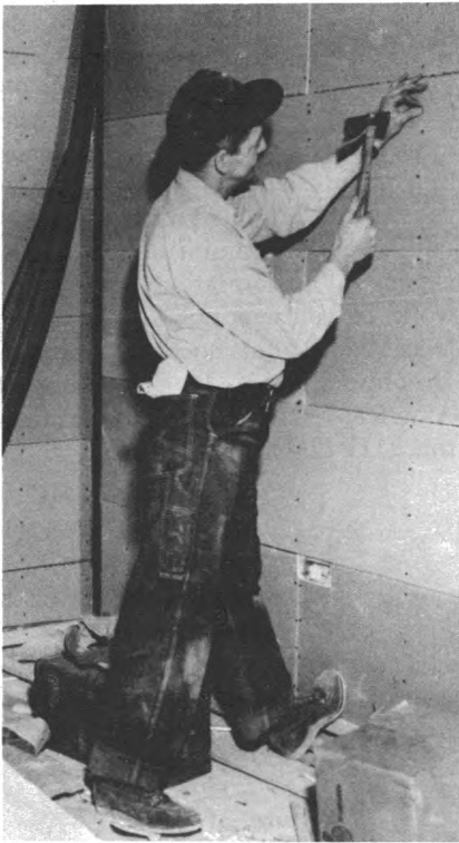
Lather nails gypsum lath to house framework.
