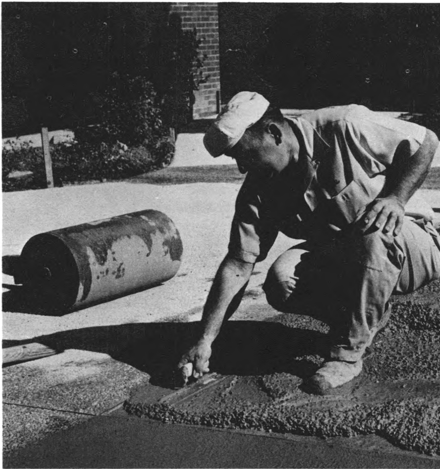
Terrazzo worker trowels top course of cement and marble chips.
