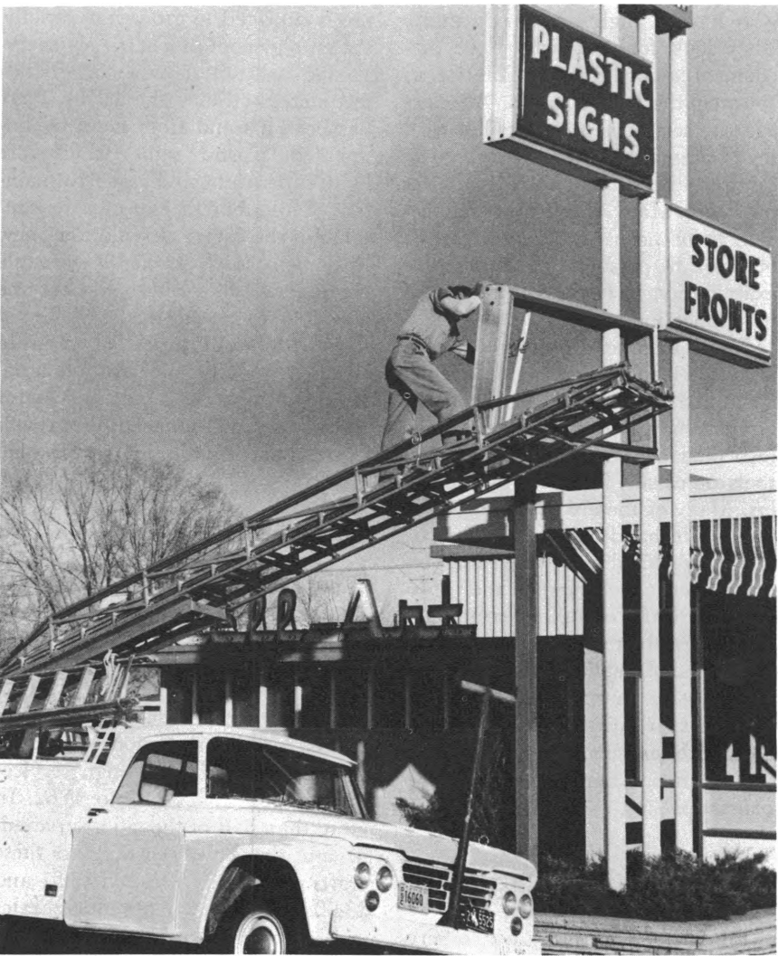
Electric sign serviceman installs lamps in illuminated plastic sign.
