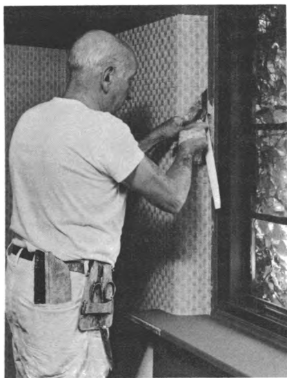
Paperhanger removes excess wall covering around window frame.
