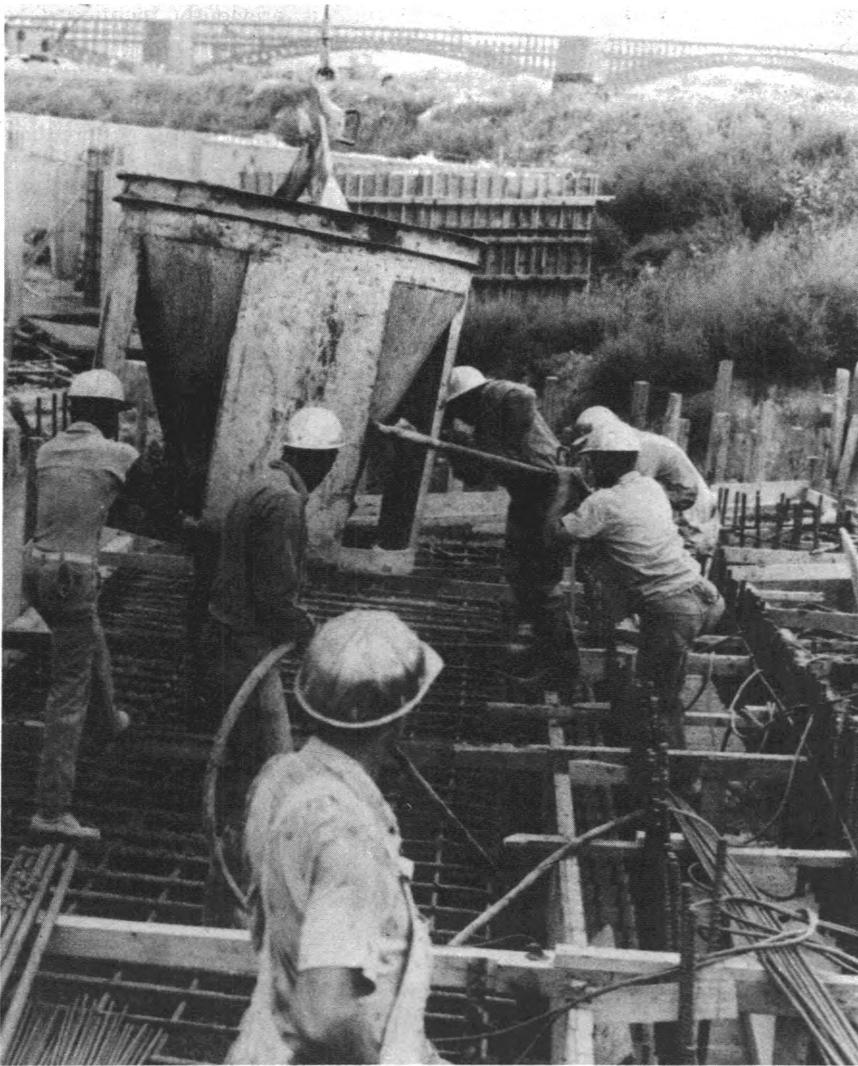
Construction crew releases concrete from bucket.
