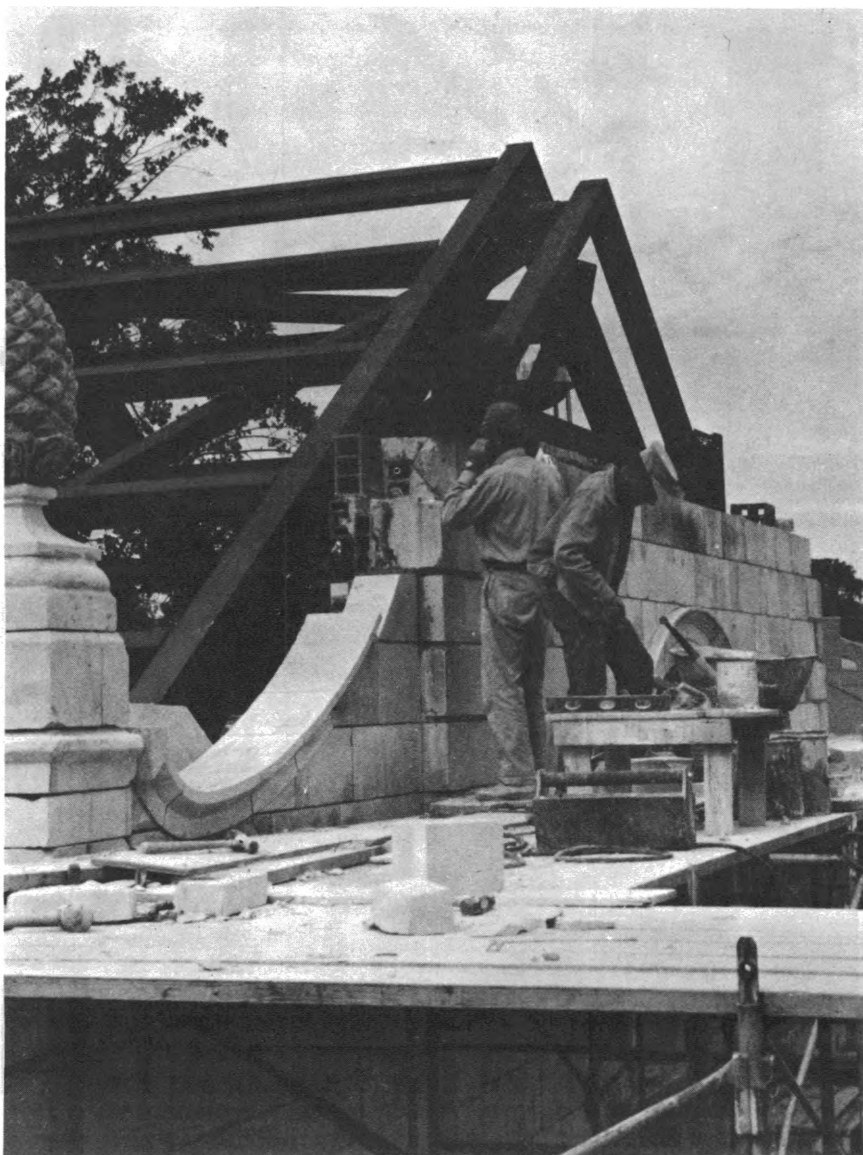
Stonemasons reconstruct old church.
