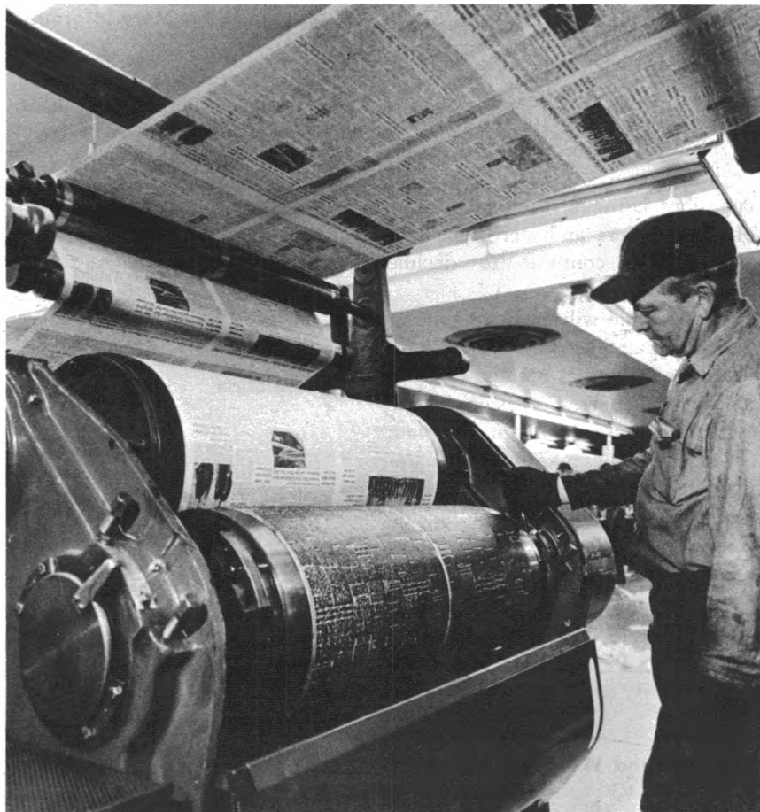
Pressman adjusts stereotype plate on newspaper press.
