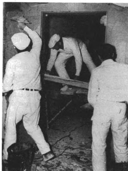
Plasterers patch surfaces around added doorway.
