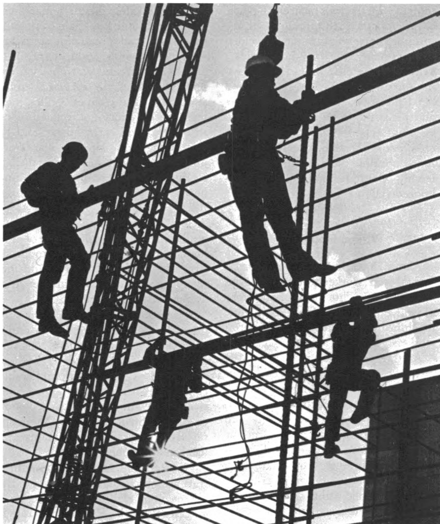
Reinforcing-iron workers (rodmen) wire steel rods in place.
