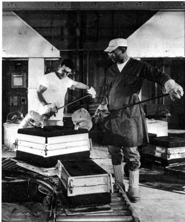
Pourers fill molds on conveyor line with molten aluminum.
