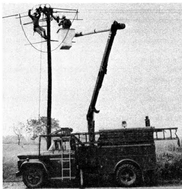
Linemen work on lines from "bucket truck."
