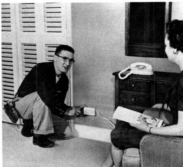
Installer mounts connecting block for telephone.
