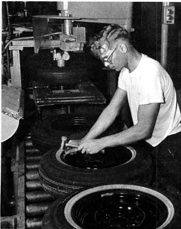
Operator places wheel weights to achieve correct wheel balance.
