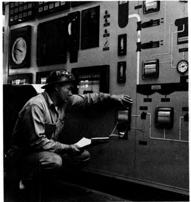
Head operator sets instrument controls that direct operation of refinery processing unit.
