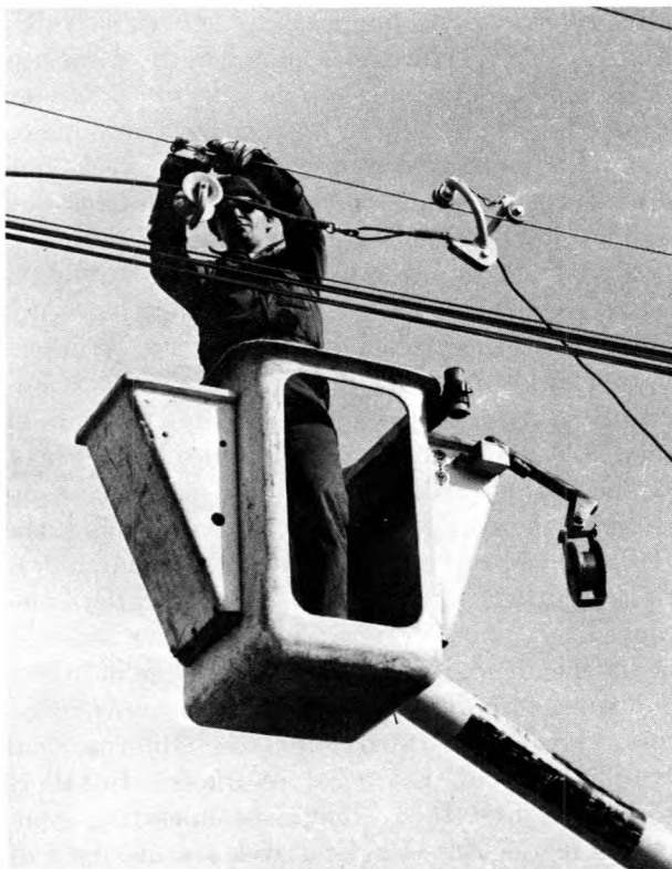
Lineman inspects cables from aerial lift.
