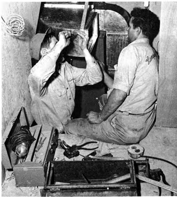
Journeyman sheet-metal worker supervises apprentice in heating-duct installation.
