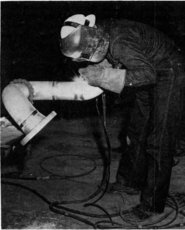
Arc welder joins sections of aluminum pipe.
