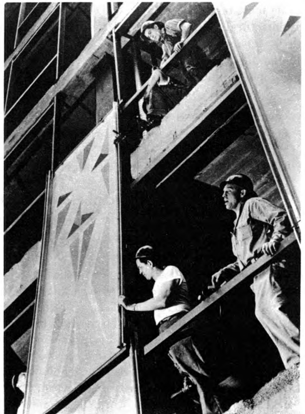
Craftsmen set ornamental stainless steel wall panel in the building framework.
