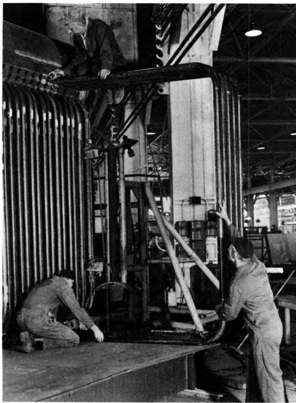
Workmen assemble wall furnace tubes for watertube boiler.
