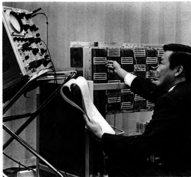
Service technician uses oscilloscope to test electronic accounting computer.
