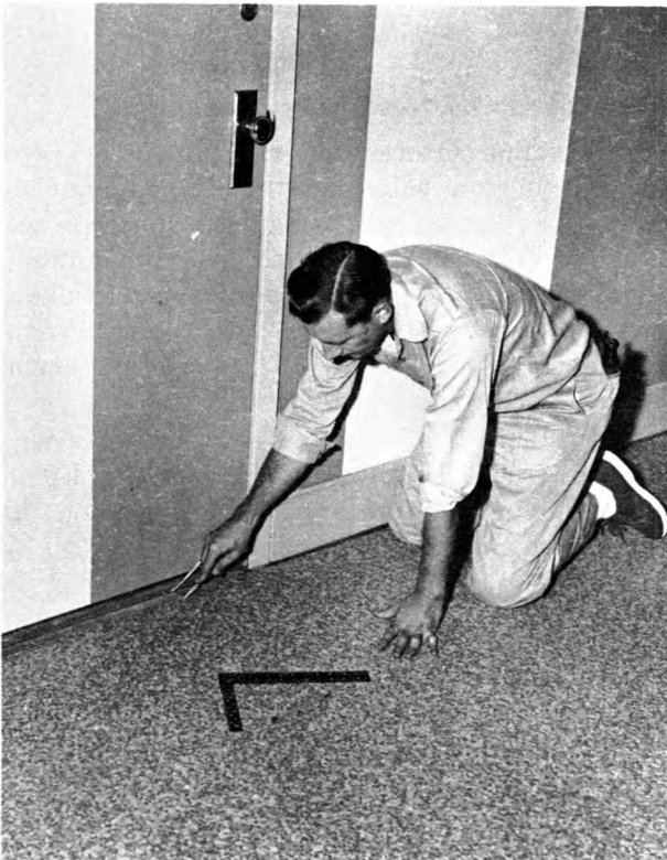
Installer marks floor covering along an irregular wall before trimming.
