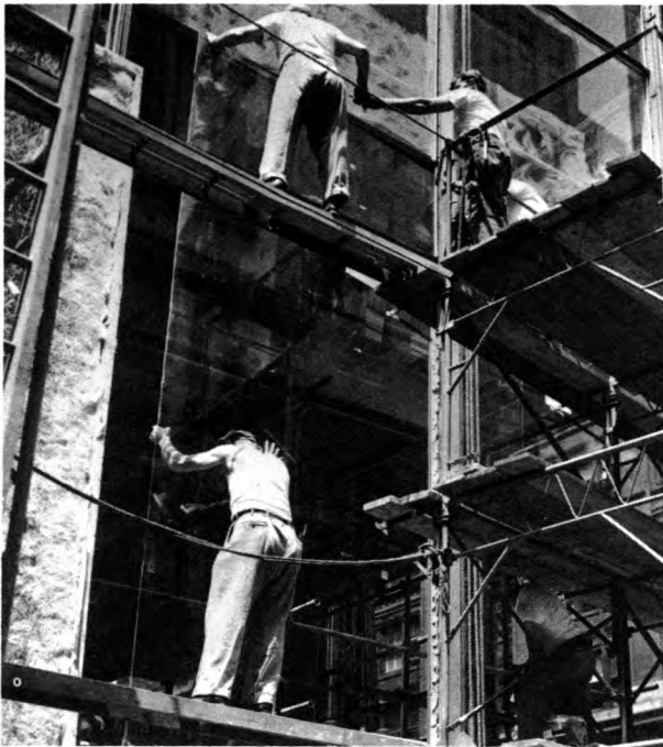
Glaziers place a glass panel in new office building.
