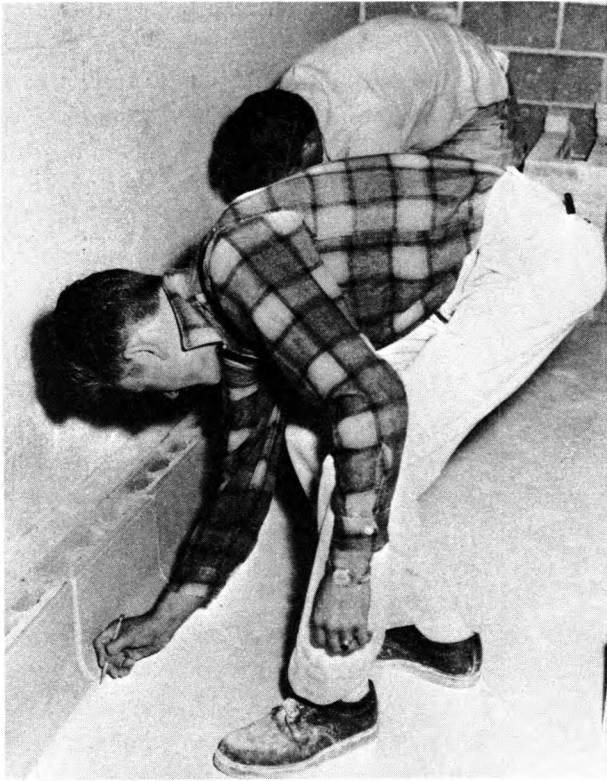
Tile setter apprentices mark off a glazed tile wall for second course.
