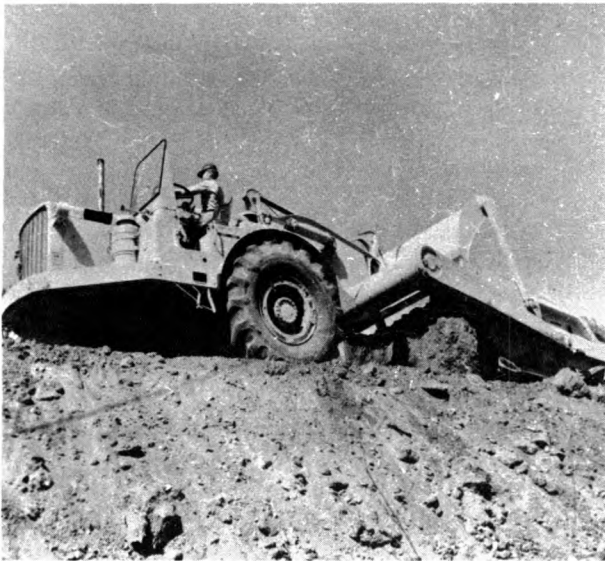
Scraper operator levels the terrain for a road.
