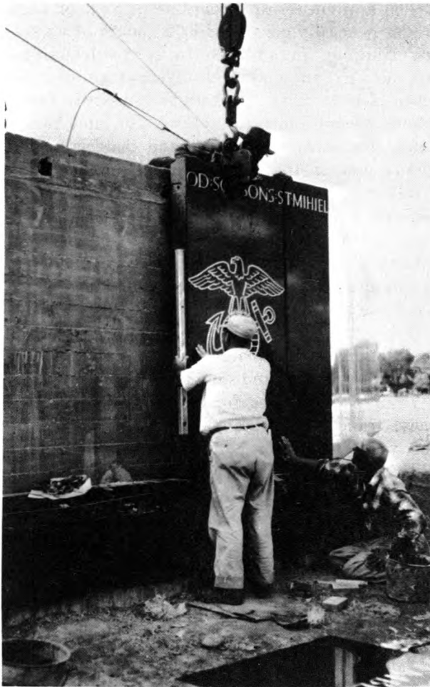
Marble setter and helpers install marble panel.
