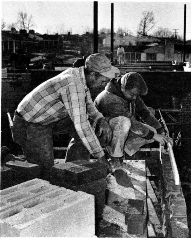
Journeyman bricklayer teaches apprentice to form a corner.
