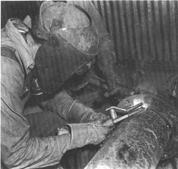
Arc welder joins flange to pipe
