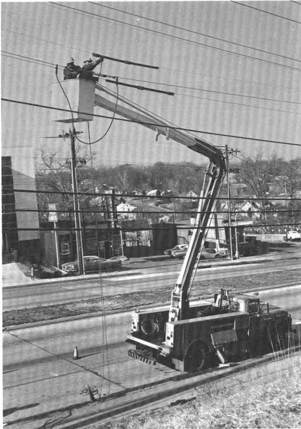
Linemen work from aerial basket to repair electric power line
