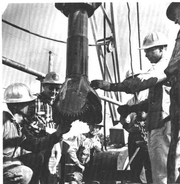
Rotary drill crew puts new drill bit into operation
