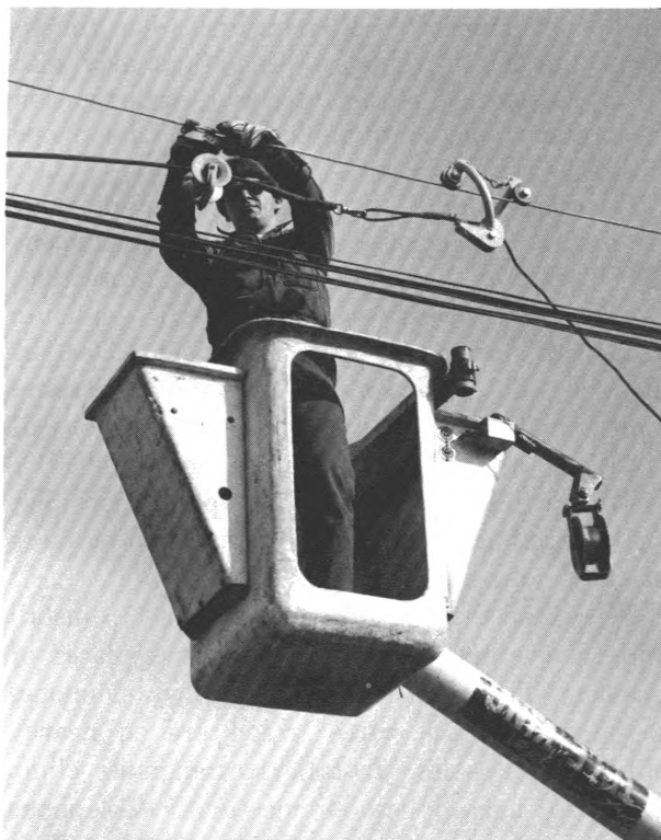
Lineman works on cable from aerial lift
