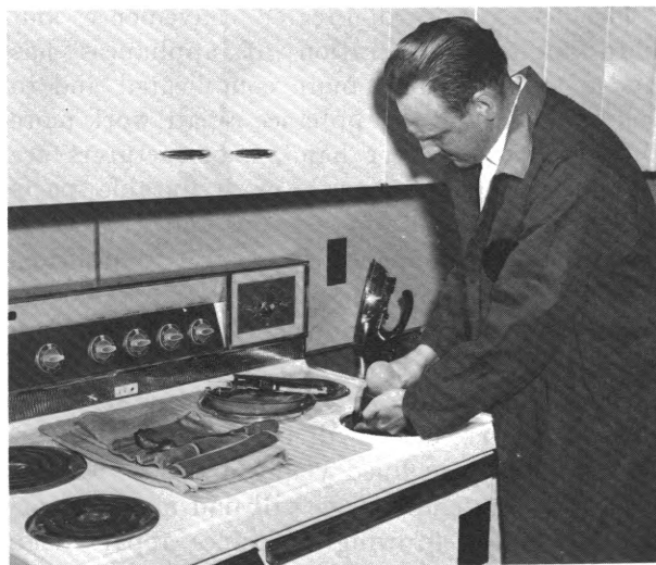
Serviceman installs surface unit in electric range
