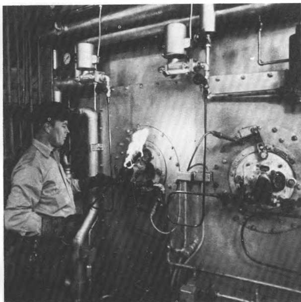
Stationary fireman lights a boiler
