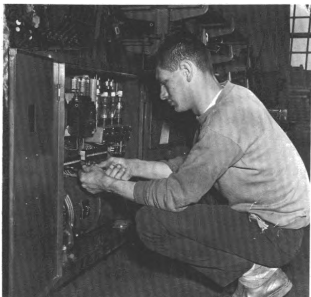
Maintenance electrician repairs connections on control panel
