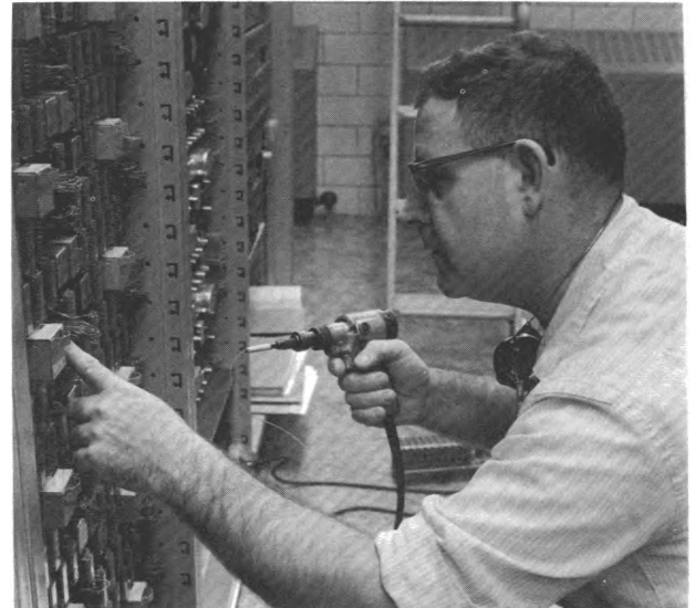
Central office installer uses wire-wrapping tool to wire equipment panel
