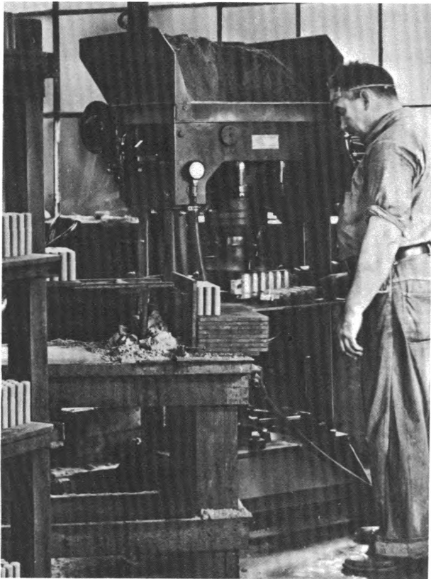
Coremaker operating machine which forces sand into hollow forms
