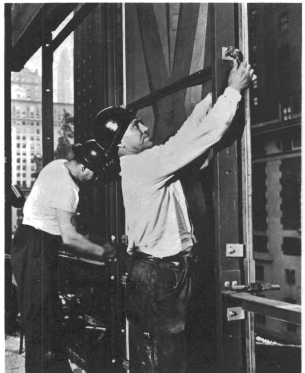
Ornamental-iron workers install stainless steel wall panels to building framework
