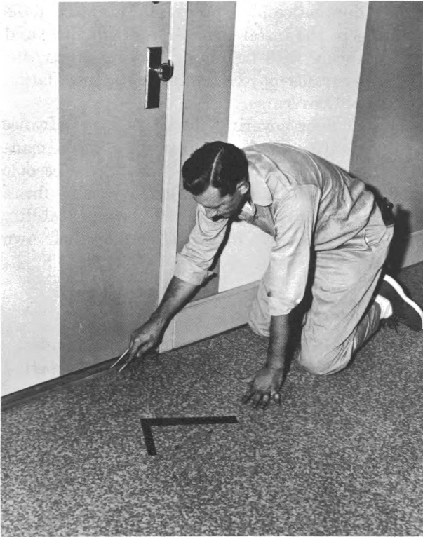
Installer marks floor covering along irregular wall before trimming
