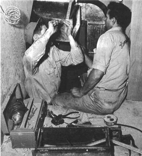
Journeyman sheet-metal worker teaches apprentice how to install heating ducts
