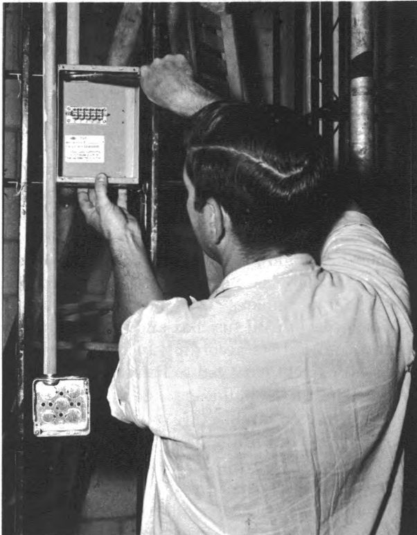
Construction electrician installs conduit and terminal boxes
