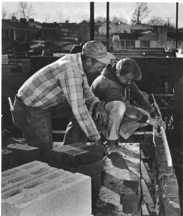
Journeyman bricklayer teaches apprentice how to form a corner
