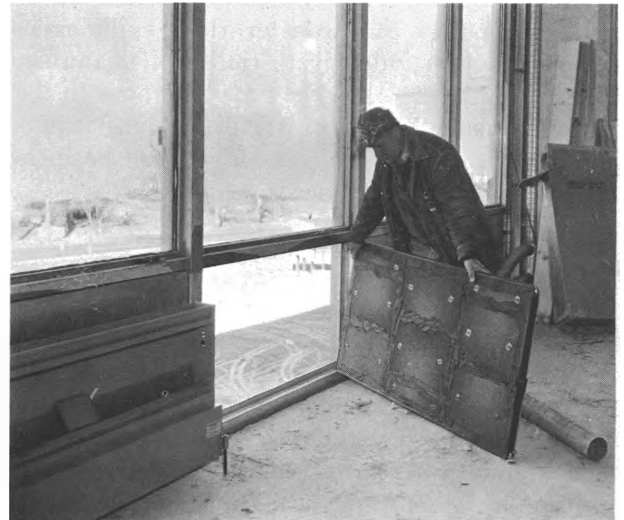
Insulation worker installs insulating panel in framework of building
