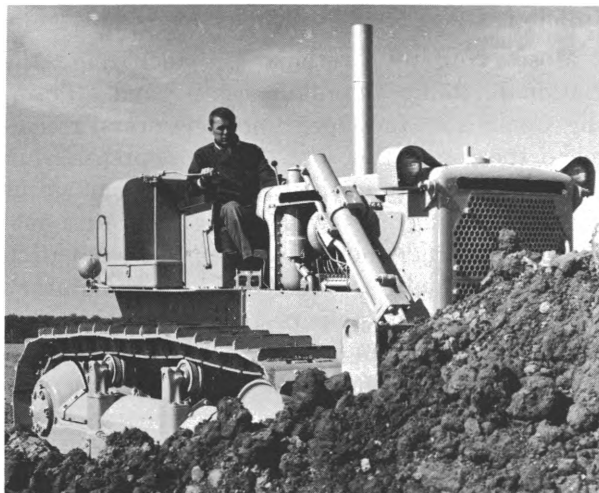
Bulldozer operator levels terrain for road
