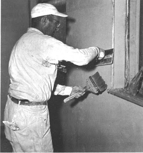
Plasterer finishes wall, using trowel and brush
