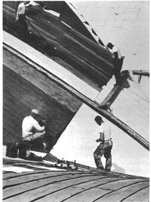
Roofers install composition roofing material on barrel-shaped roof
