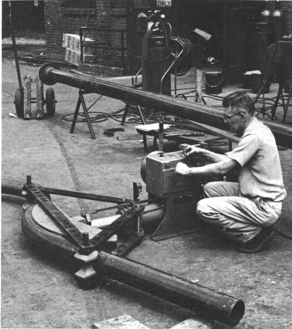
Pipefitter bends pipe with hydraulic pipe bender
