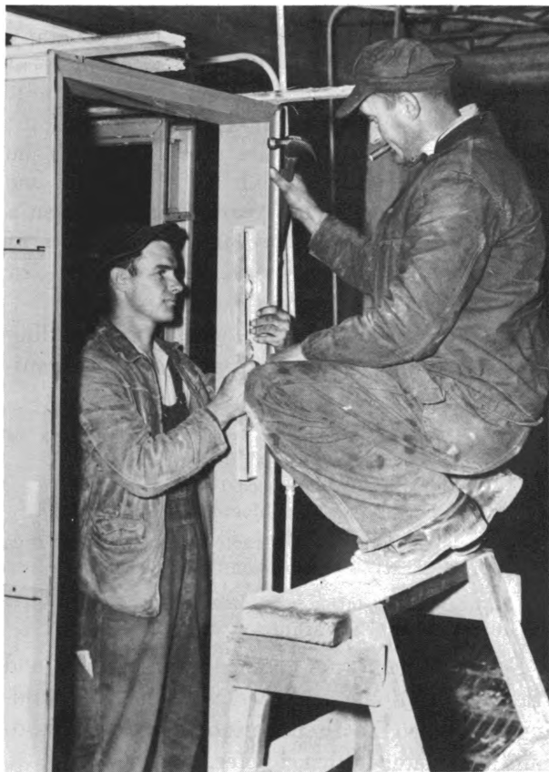
Journeyman carpenter shows apprentice how to line up doorframe
