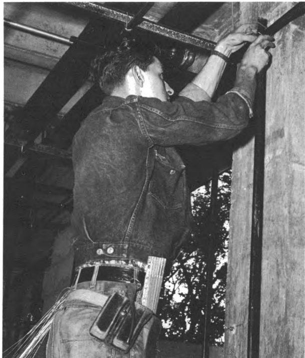
Lather installs metal furring used to support lath
