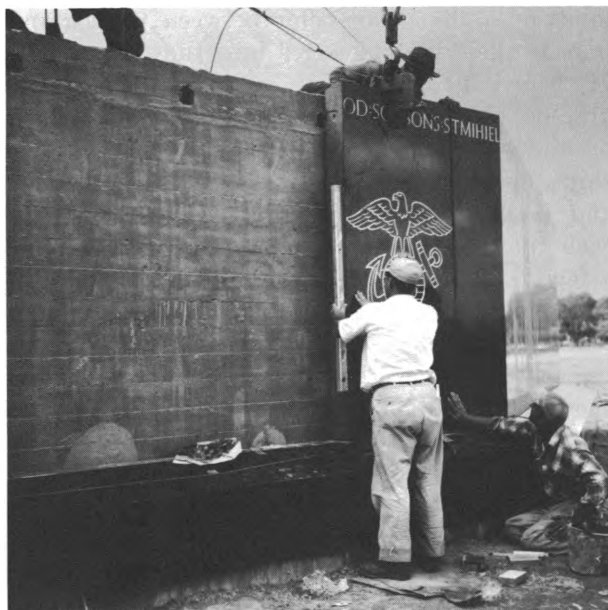
Marble setter and helpers install marble panel
