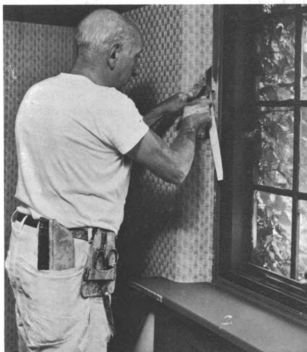
Paperhanger removes excess wall covering around window frame
