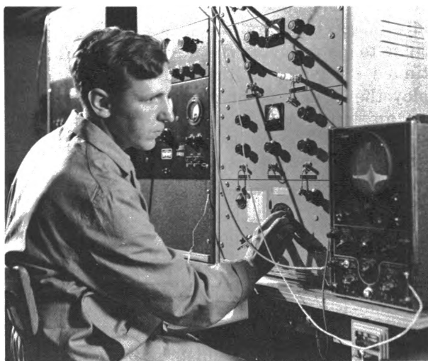
Physicist using microwave spectroscopy to measure atom masses.
