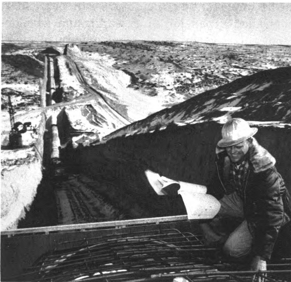
Civil engineer inspecting reinforcing steel used in a river basin project.
