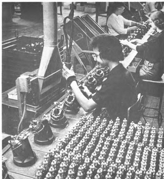
Assembler soldering connections on automobile heater motor
