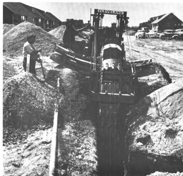
Operating engineer operating a trenching machine.
