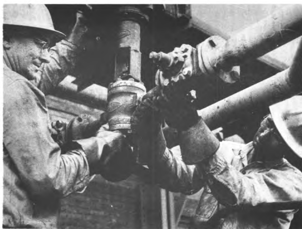
Pipefitters installing a control valve in a refinery.
