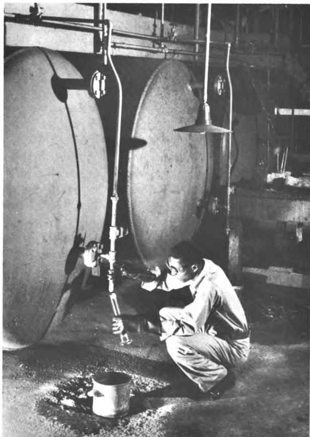
Chemical operator drawing off samples of a chemical for testing in the laboratory.
