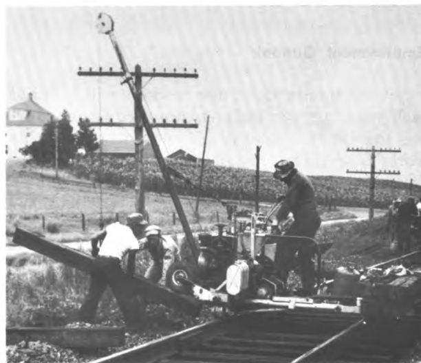
Track workers use roadway machines to speed replacing worn railroad ties.
