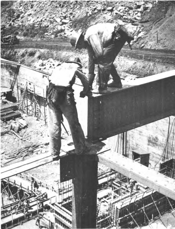
Structural-iron workers erecting structural steel framework.
