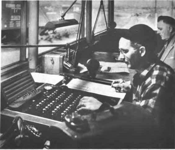
The towerman routes cars in a freight yard by throwing switch with the push of a button.
