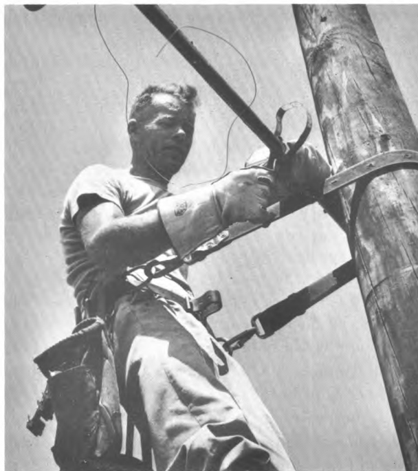
Lineman on pole secures wire with a metal strap.
