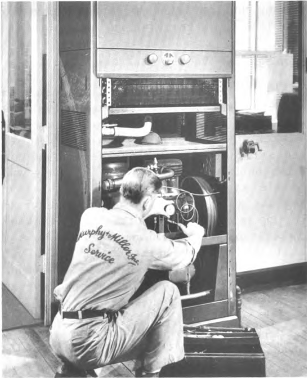
Mechanic adjusting an air-conditioning unit.
