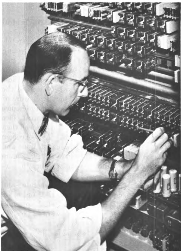
Framemen connect the thousands of pairs of wire that come into the central office from lines and cables.
