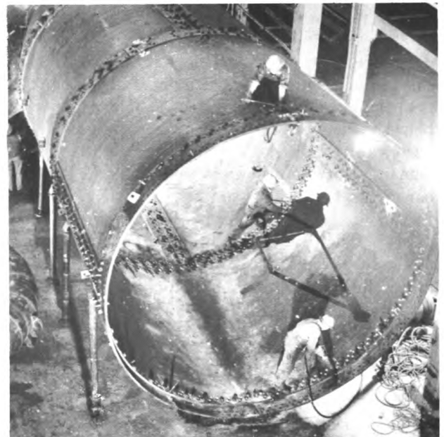
Boilermakers assembling units made of heavy steel plate.
