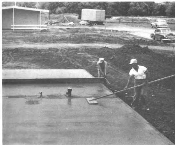
Cement finisher smoothing house slab after helpers have leveled it.
