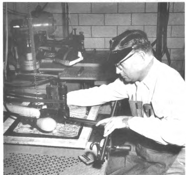
Photoengraver cutting away metal from nonprinting areas of a plate.
