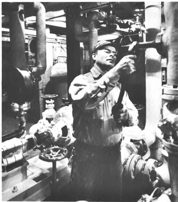
Stationary engineer adjusting a valve.
