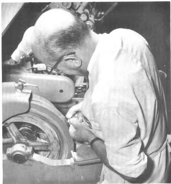
Optical machanic (finisher) hand beveling a nearly completed lens.
