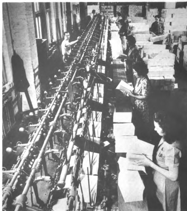
Bindery workers assembling material on gathering machine.
