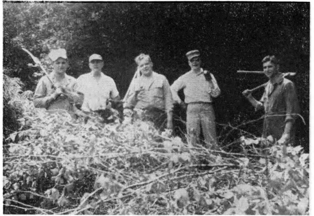
FIGURE 12.—“Burma Drive clearing detail” at Kirkmere Home Owners, Youngstown, Ohio.
