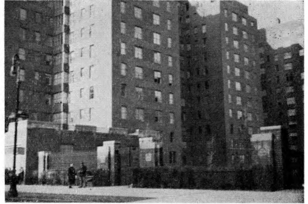
FIGURE 25.—Hillman Houses (all-the-way project of the Amalgamated group), in lower Manhattan, N. Y.
