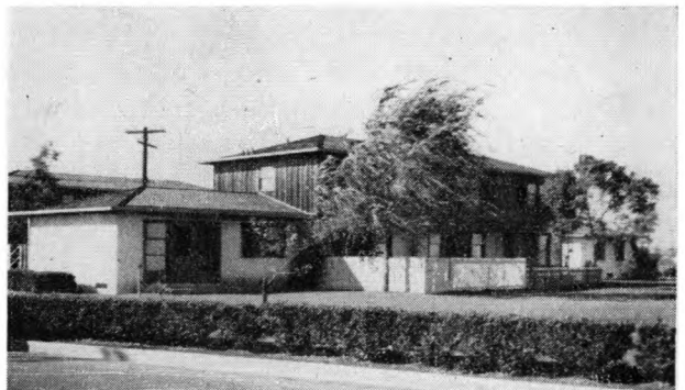
FIGURE 29.—Views at Victory Park, mutual project of Mutual Housing Association of Compton, Calif.
