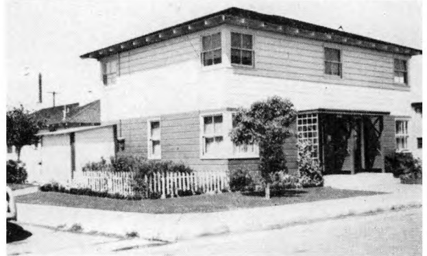
FIGURE 28.—Views at mutual project of Alameda (Calif.) Mutual Homes Corp.
