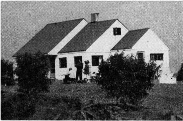
FIGURE 14.—Upper: House built by exchange-of-labor method in prewar co-venture project at Penn-Craft, Pa. (stone quarried on site). Lower: House built by member's own labor in postwar co-venture project at Penn-Craft, Pa. (cinder blocks made by members).
