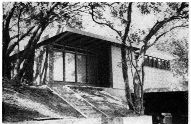
FIGURE 13.—House built by member's own labor, Hermits Glen co-venture project, Los Angeles, Calif.
