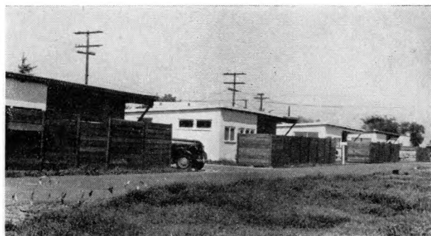
FIGURE 16.—Side view of Bay Area Housing Group's co-venture project, showing dwellings one behind the other on same lot, and fenced service yards, Culver City, Calif.
