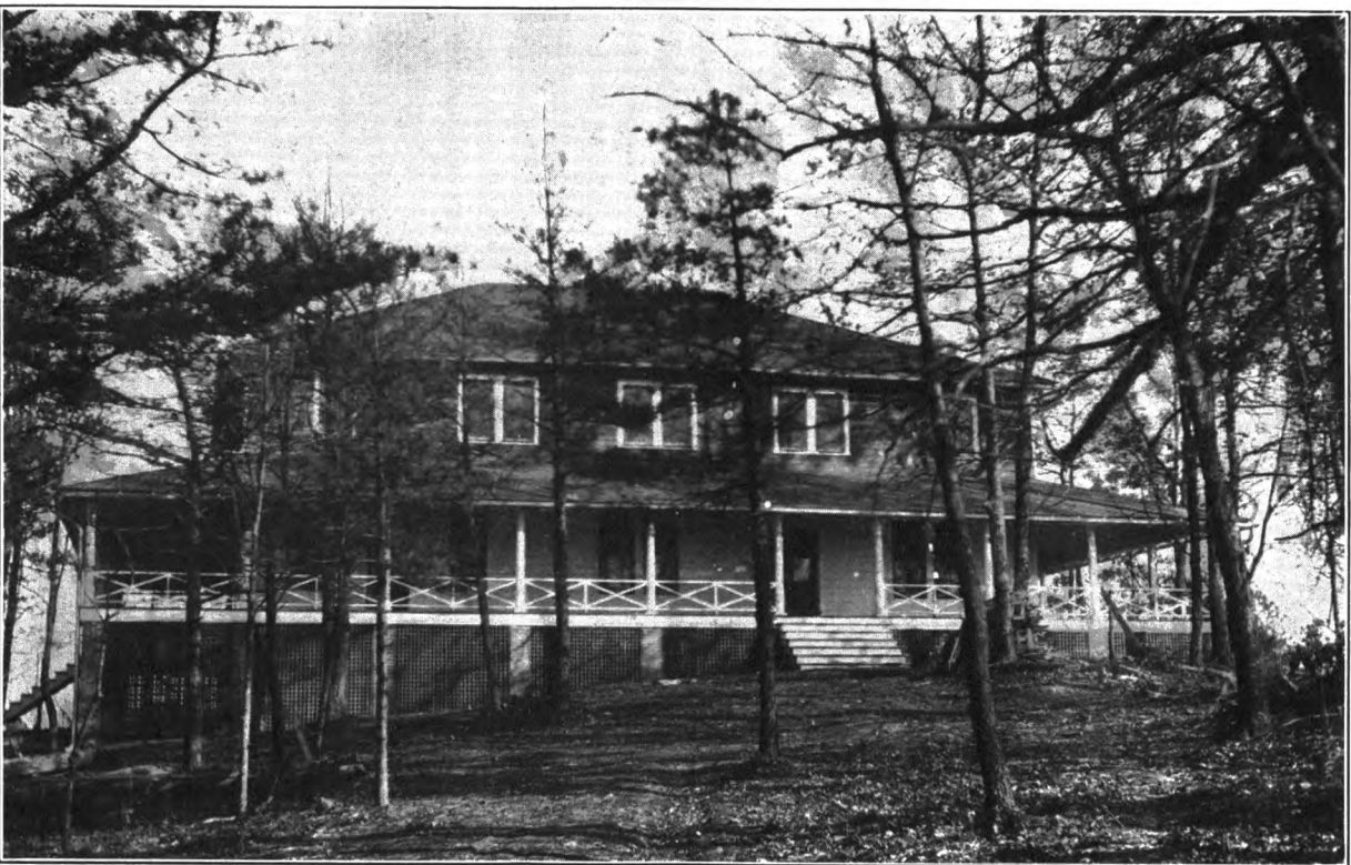
FIG. 16.—Recreation lodge of Brotherhood of Railway Clerks' locals on Southern Railway System
