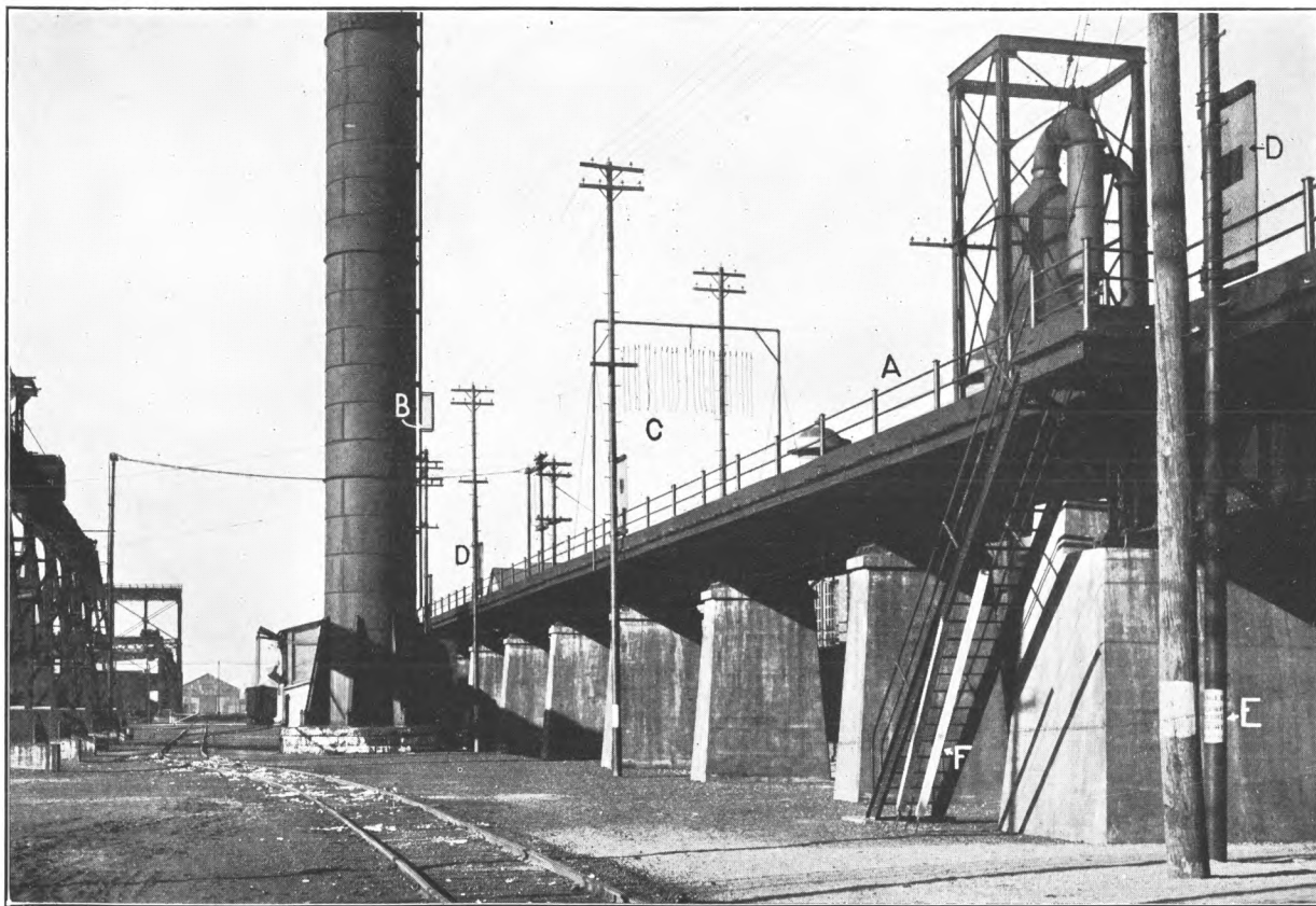
PLATE 20.—YARD TRESTLE, WITH VARIOUS SAFETY DEVICES.
