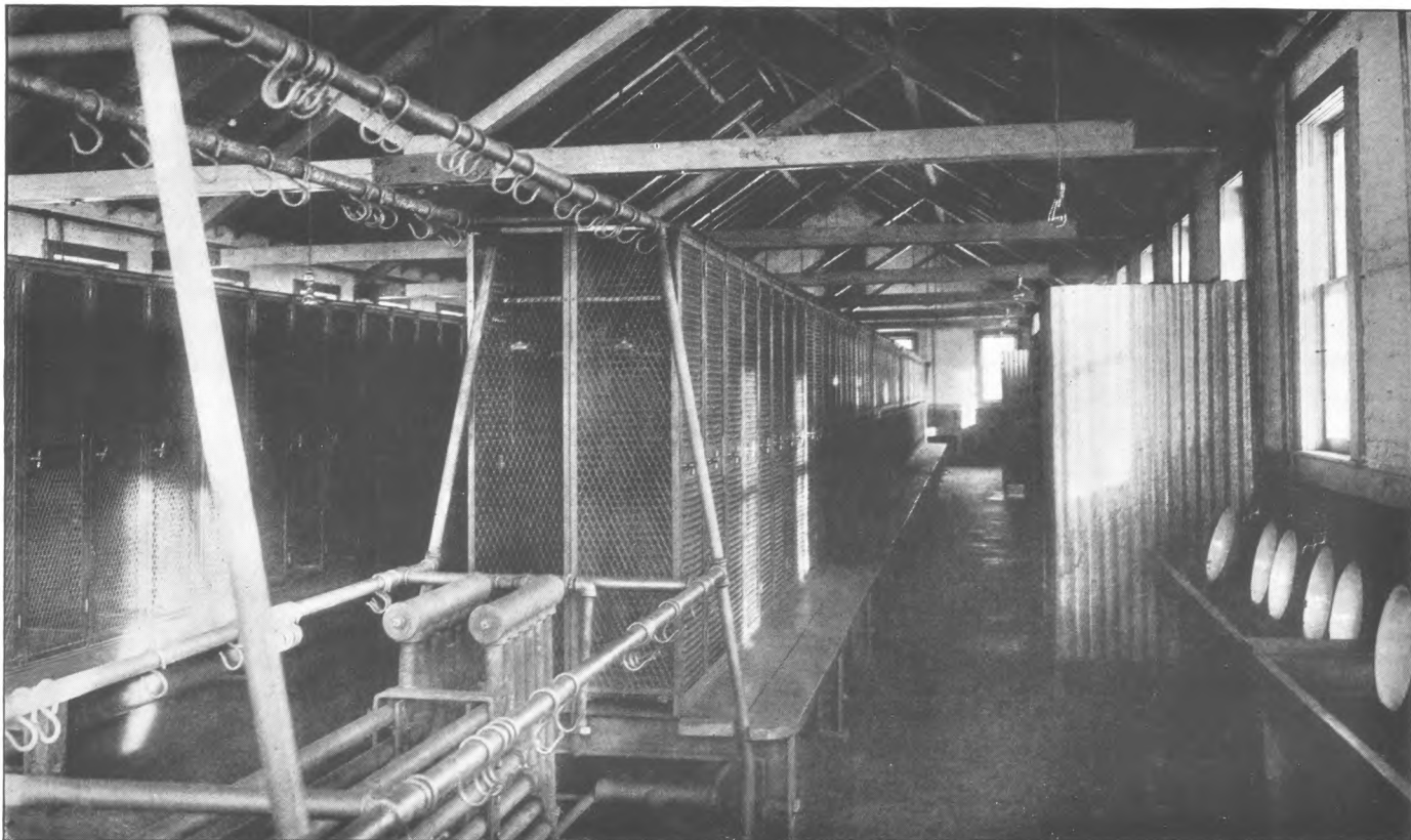
PLATE 15.—INTERIOR OF WASH AND CHANGE HOUSE; BASINS IN TROUGH, SHOWERS BEYOND; STEAM PIPES UNDER LOCKERS; BENCHES; S-SHAPED HOOKS ON STEAM PIPES FOR DRYING CLOTHING.
