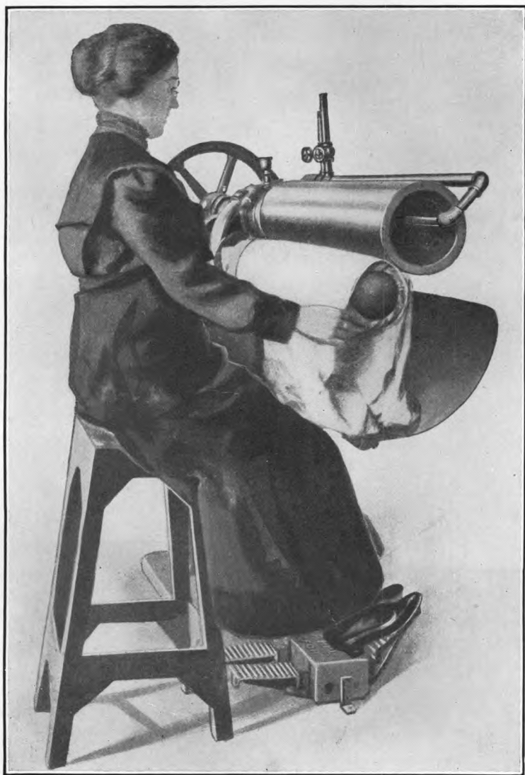
PLATE 2.—BODY IRONER EQUIPPED WITH PNEUMATIC TREADLE.
