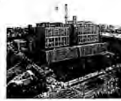
U.S. Capitol Power Plant Washington, DC
