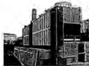
U.S. Capitol Power Plant Washington, DC
