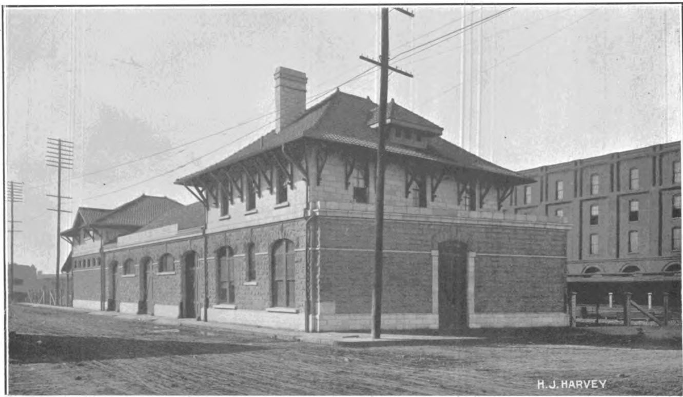
STABLE AND TOOL HOUSE —Erected 1910.
