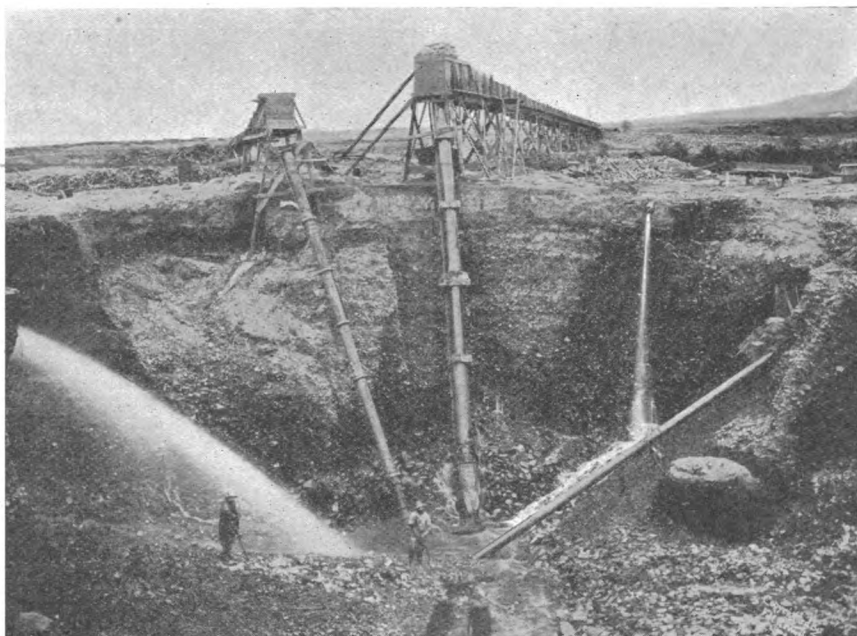
HYDRAULIC LIFT, USED IN FLAT COUNTRY; WATER UNDER PRESSURE —Photo by Frank H. Nowell
