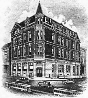
AMERICAN NATIONAL BANK BUILDING.
