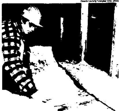
Manufacture and installation of insulation are booming.
