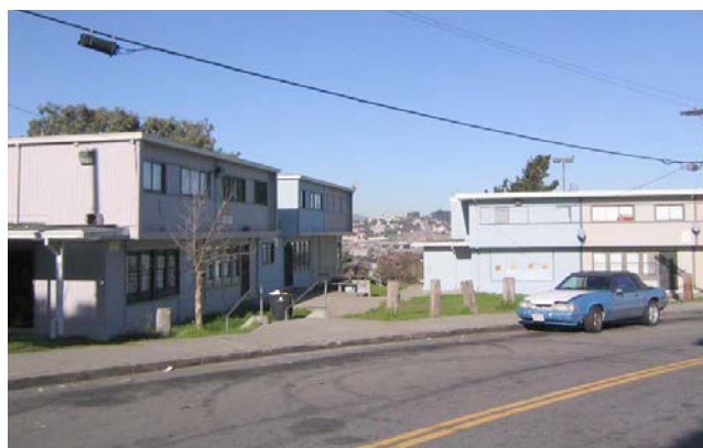
Current housing units at Hunters View Photo courtesy of John Stewart Company
