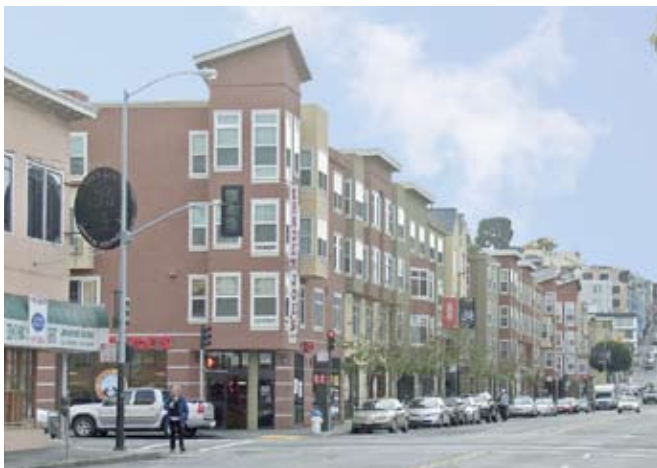
North Beach Place is a HOPE VI project built in 2004 in San Francisco
