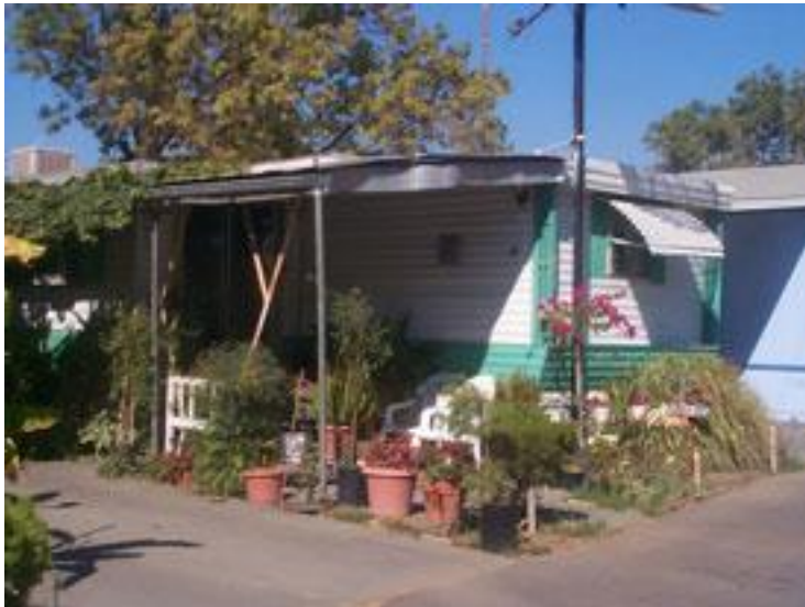
One of the existing mobile homes - in good condition
