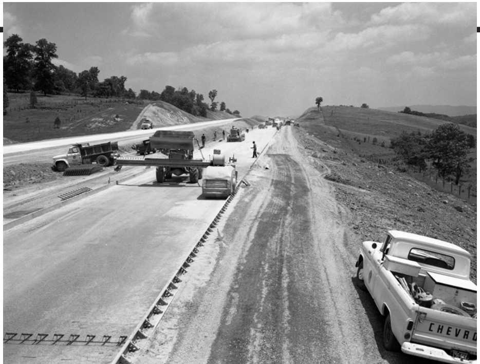
Interstate 81 under construction in Botetourt County, Va., in June 1964.
