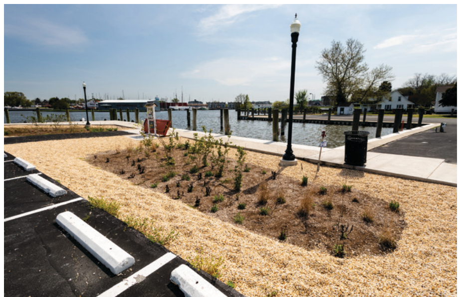
A rain garden at Long Wharf Park captures and filters stormwater pollution before it reaches the Choptank River in Dorchester County, Md.
