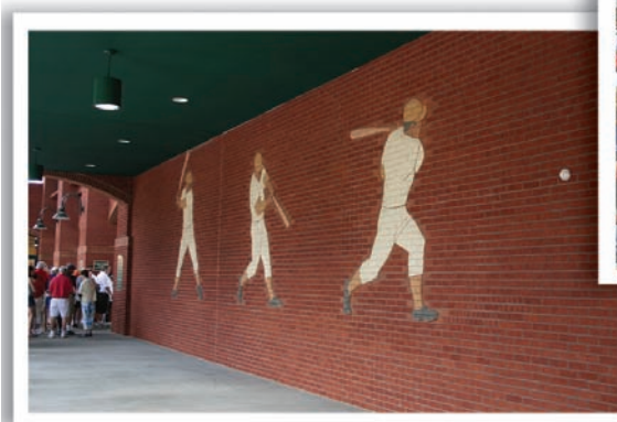
NewBridge Bank Park — Greensboro, N.C.
