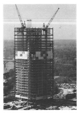
A white painted steel beam with the American flag attached is shown approaching the northwest corner of the new building where its installation, known as topping-out, will symbolize the completion of structural steel work.
