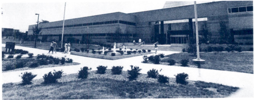
Enrollment is up at WACC, due to the new Advanced Technology and Health Sciences Center---a futuristic educational facility.
