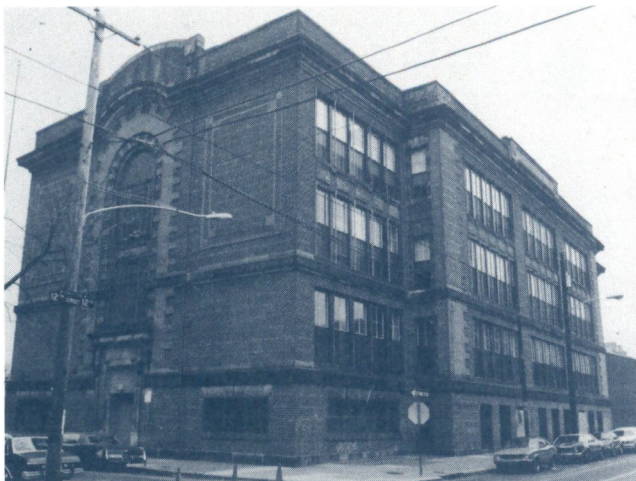
Hawthorne School before the renovation. It is one of a group of Philadelphia schools certified as historic, and its original classroom doors and blackboards were preserved.
