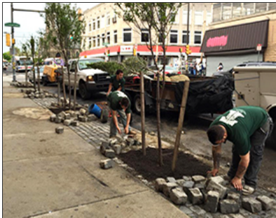
Tree planting near the intersection of Germantown and Cheltenham Avenues in Philadelphia helps beautify a busy commercial corridor. Photo Credit: Aine Doley
