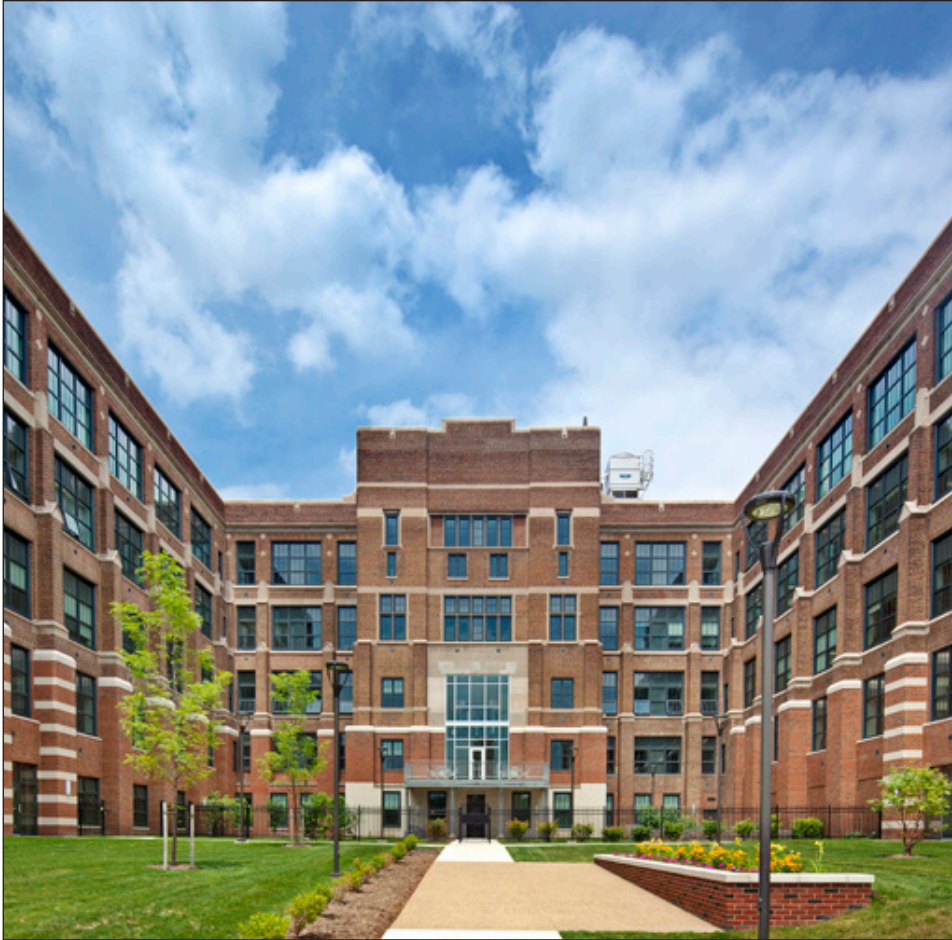
South Hills Retirement Residence, a 106-unit building for residents 55 and over in Pittsburgh, was substantially rehabilitated with financing from the PHFA and other sources.
