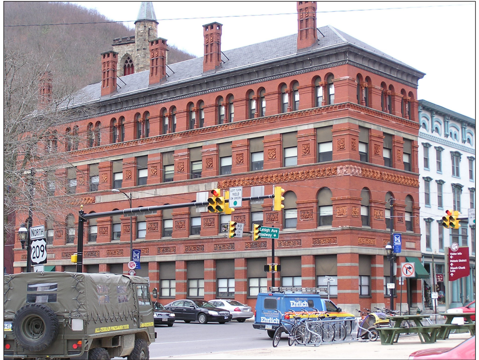
The historic Lehigh Coal and Navigation Building, located in the central business district in Jim Thorpe, PA, is an example of a rehabilitation and preservation project financed with the assistance of the Pennsylvania Housing Finance Agency. The building provides 27 subsidized rental units for older people.
