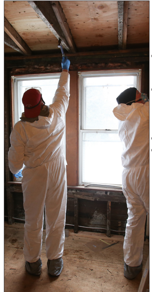
Credit: Bennett Raglin/AP Images for Rebuilding Together
