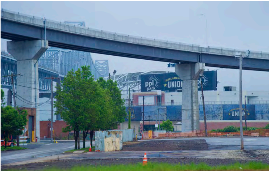
▶ New ramp from the Commodore Barry Bridge to Chester, PA, including PPL Park, home of the Philadelphia Union professional soccer team
