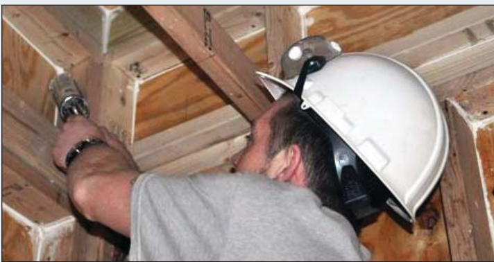
A trainee practices air sealing at the Knight Green Jobs Training Center.
