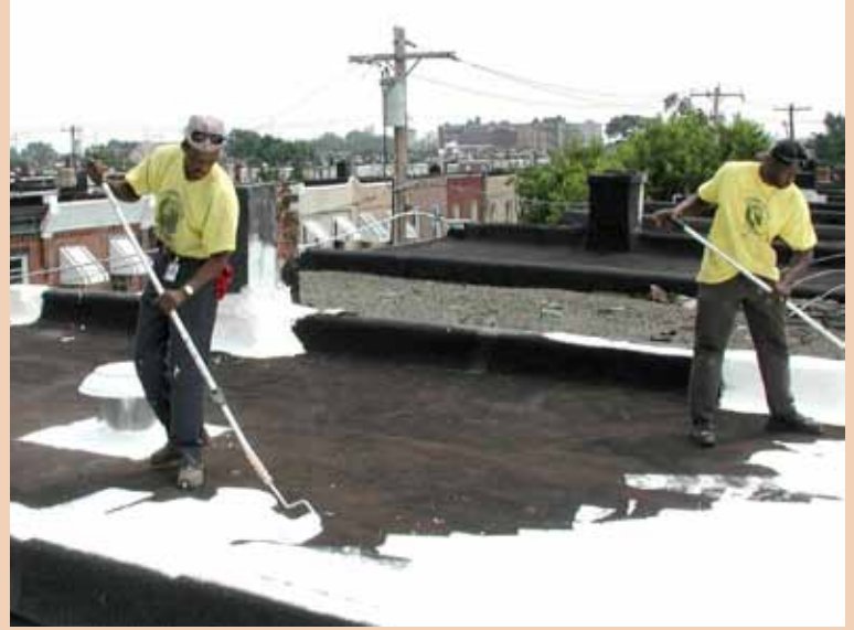
Energy Coordinating Agency (ECA) employees air-seal and insulate a roof with spray foam and then coat the roof with a white paint that is durable and waterproof and provides a reflective coating.
