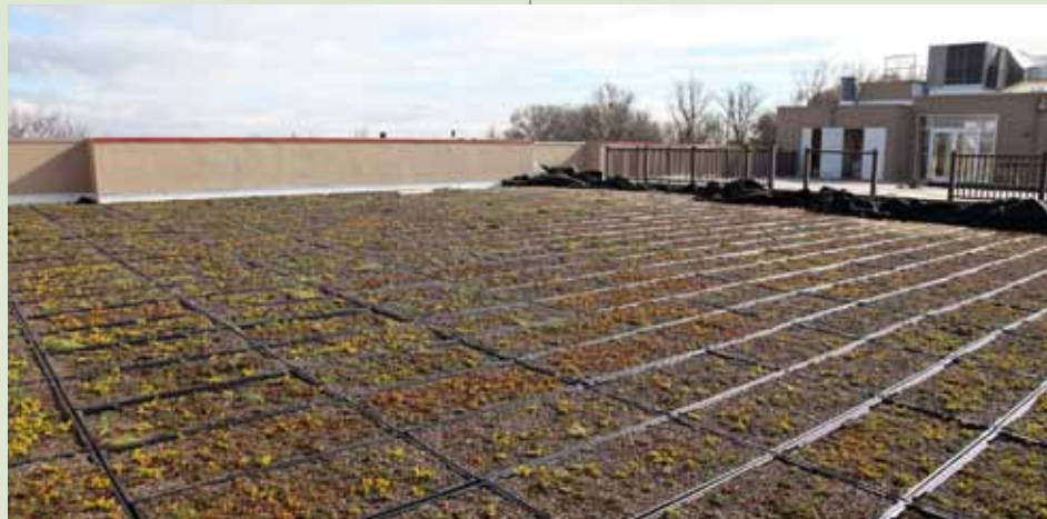
This green roof atop the Philadelphia Housing Authority's Warnock Village senior building is one of the energy-efficiency improvements made by the Philadelphia Housing Authority since the agency started working with a Drexel University research and advisory team.
