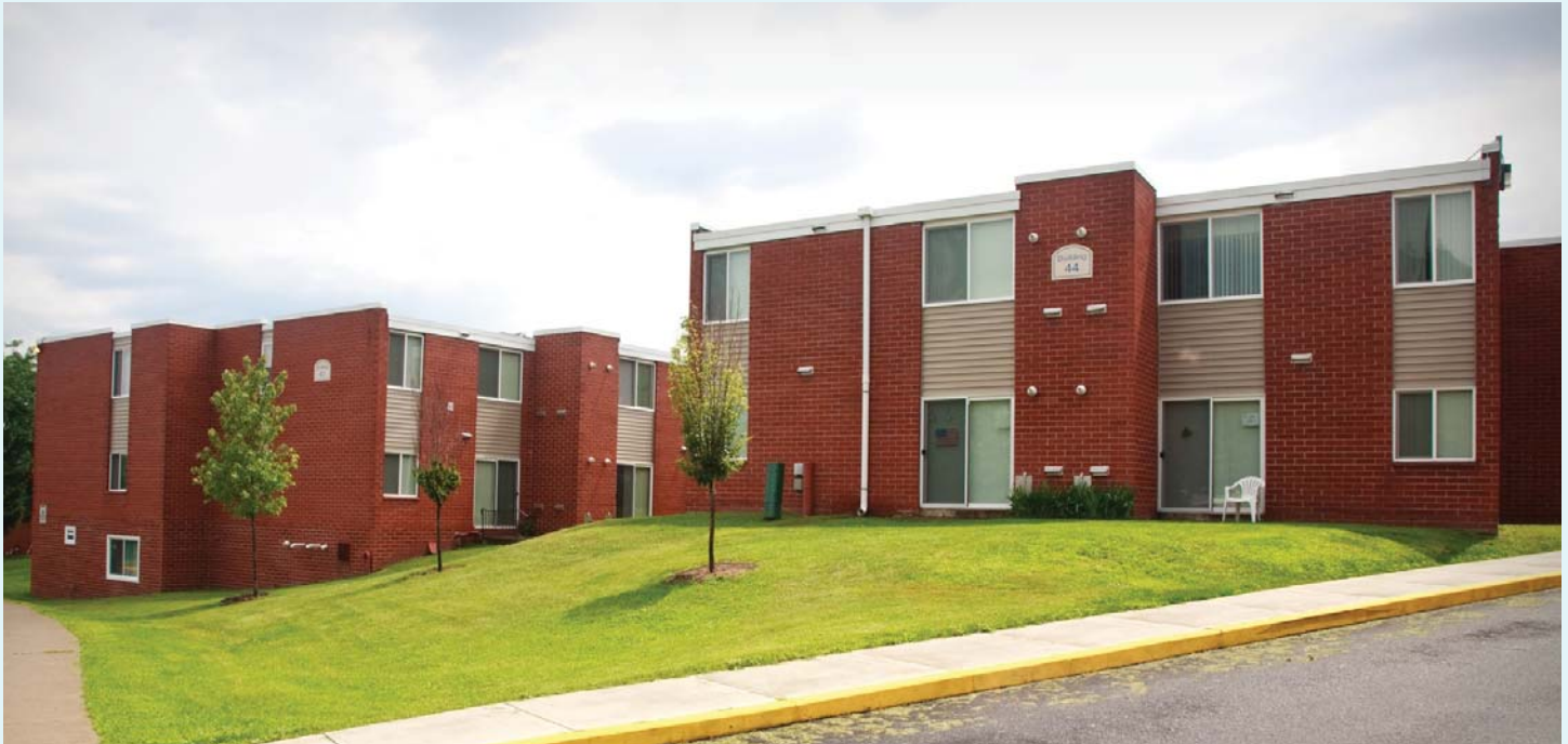
The Skyview Park Apartments in Scranton, PA, have been renovated with capital improvements that reduced energy use and conserved water.
