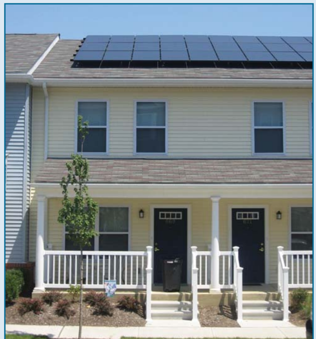
A $16.8 million low income housing tax credit investment from JP Morgan Chase helped finance the rental units shown above as part of an 11-phase HOPE VI redevelopment plan in Camden, N.J. The project, Carl Miller Homes, was completed in December 2008 and used solar panels to help meet power needs. Michaels Development was the developer, and the Camden Housing Authority provided significant additional funding.
