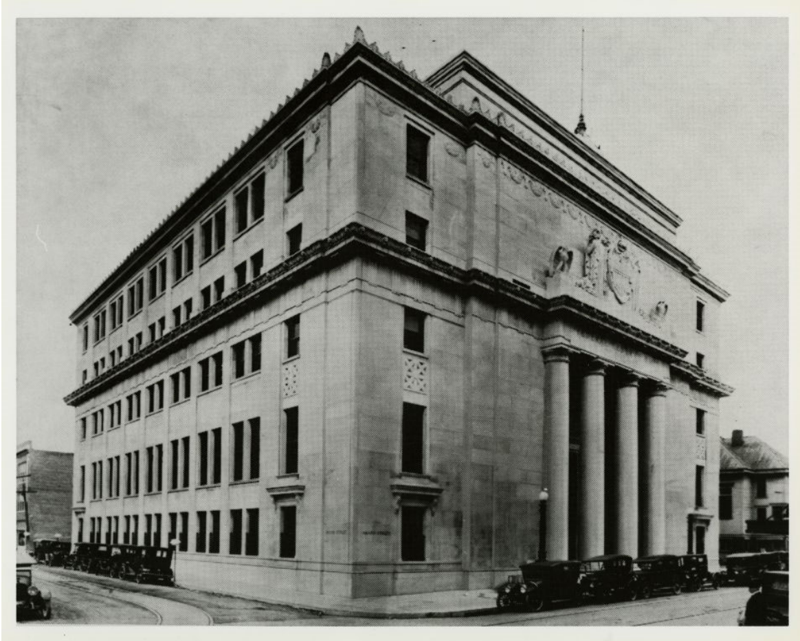
Figure 11 – Original Building on Wood and Akard Street Site
