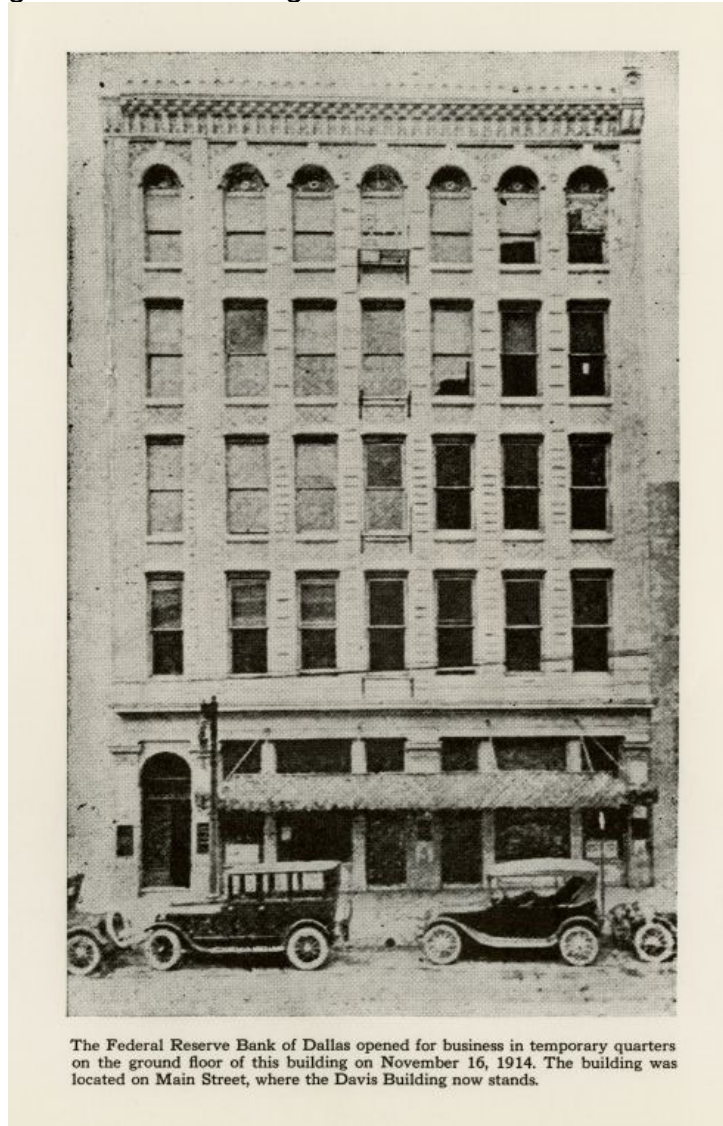
Figure 5 – Building in Which Bank Opened for Business
