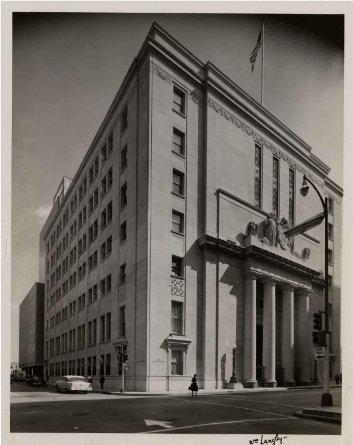
Figure 1 – Head Office Building
