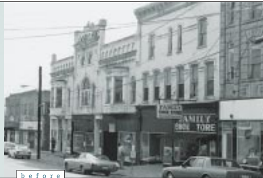
The Main Cross Project Elderly Housing/Commercial Incubator Mt. Sterling, Kentucky (see also front page photo)
