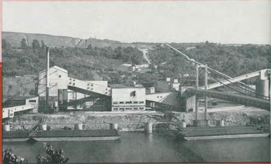
Coal processing plant on the Monongahela
