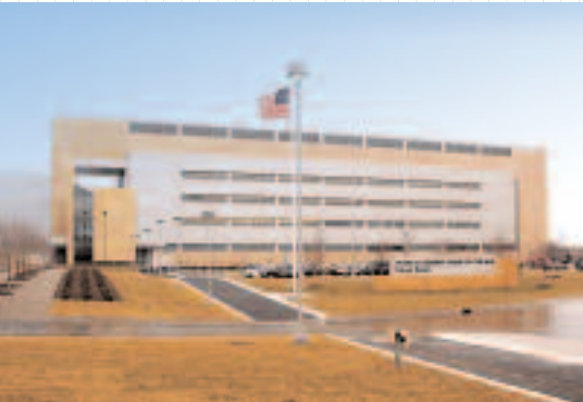
One of the Bank’s 2005 highlights was the December opening of the new Detroit Branch building.
