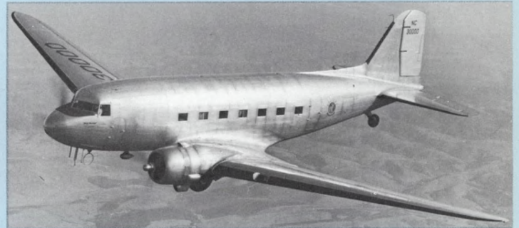
DC-3: 1936; 21-28 pass.; 170-185 mph; 13 tons; short range DC-2 (similar to DC-3, but smaller): 1934; 14 pass.; 175 mph; 10 tons; short range
