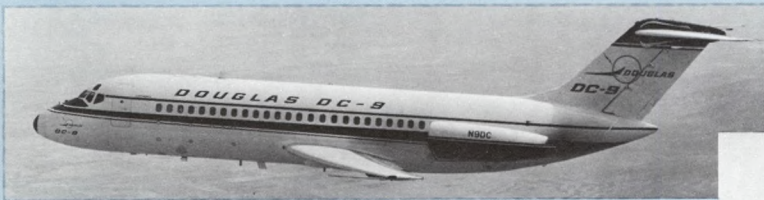
DC-9 series: 1965 to date; 56-115 pass.; 550 mph; 39-45 tons; short range
