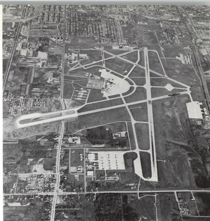
Milwaukee's Mitchell Field—extension of jet runway required a tunnel for highway traffic
