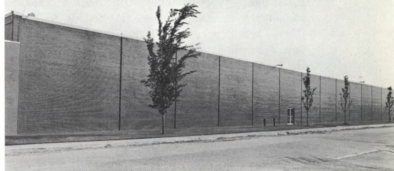
Windowless factory simplifies construction and internal arrangements
