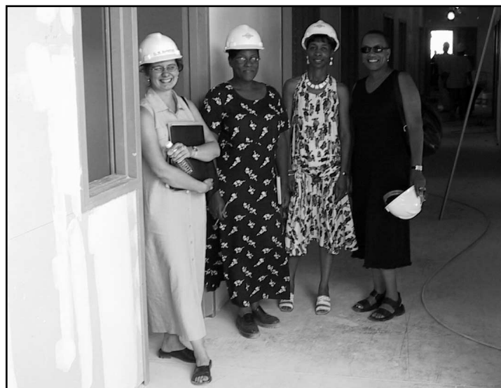
Gabriella DiFilippo, Illinois Facilities fund and Kim Jackson, Sheila Barber and Stanley Merriwether of Lawndale Christian Development Corporation review the construction of a Jubilee Family Resource Center in Lawndale.
