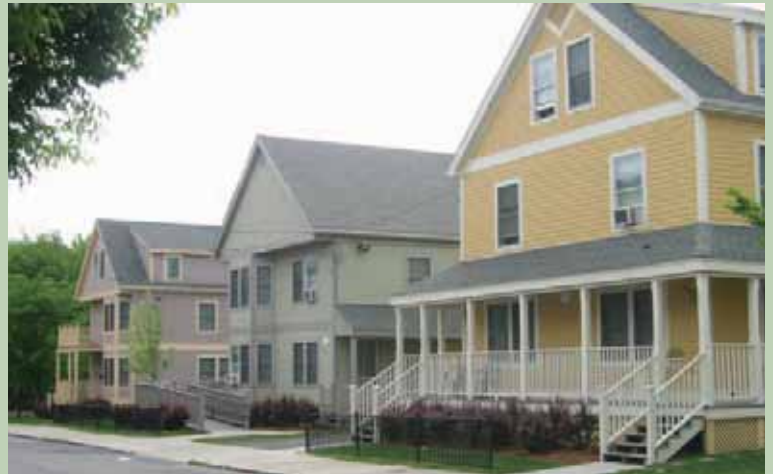
Energy efficient homes on Ellington Street in the Erie-Ellington area of Dorchester built in 2000. Photographs in this article are from the Heart of the City database, www.heartofcity.info .
