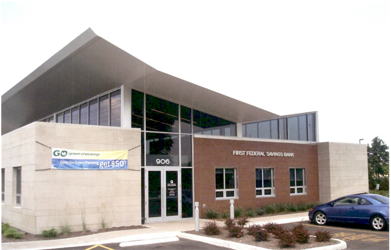
First Federal Savings Bank in Mishawaka, Indiana, uses wind turbines, geothermal heating and cooling systems, and solar panels to help meet its own energy needs. Natural lighting not only reduces energy consumption; it also provides a positive environment for employees and customers. The bank opens its doors to schools and others to show how, according to First Federal President Richard E. Belcher, "One bank can make a difference. One person can make a difference."
