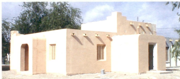
Omni's prototype of EPS foam construction shows architectural adaptability.
