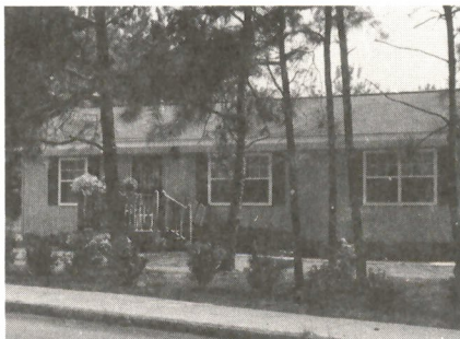
This 9-unit subdivision was developed by Progressive Redevelopment, Inc., Atlanta, and combined a small grant from a local nonprofit organization with an A&D loan from SERV. Permanent financing was provided by the Atlanta Mortgage Consortium.
