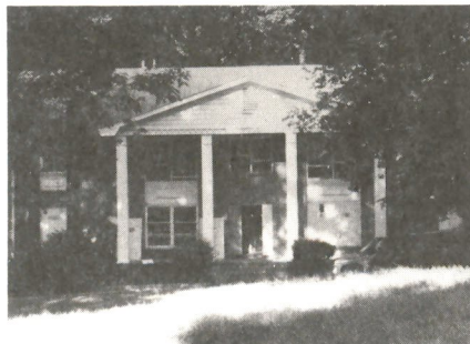
Congregations for Affordable Housing, a nonprofit organization, is rehabilitating this 28-unit co-op in Decatur, GA, with funds from a state housing trust fund, the Dekalb County Housing Authority, a local S&L, and SERV. Permanent financing will be provided by the Atlanta Mortgage Consortium and the National Co-op Bank.
