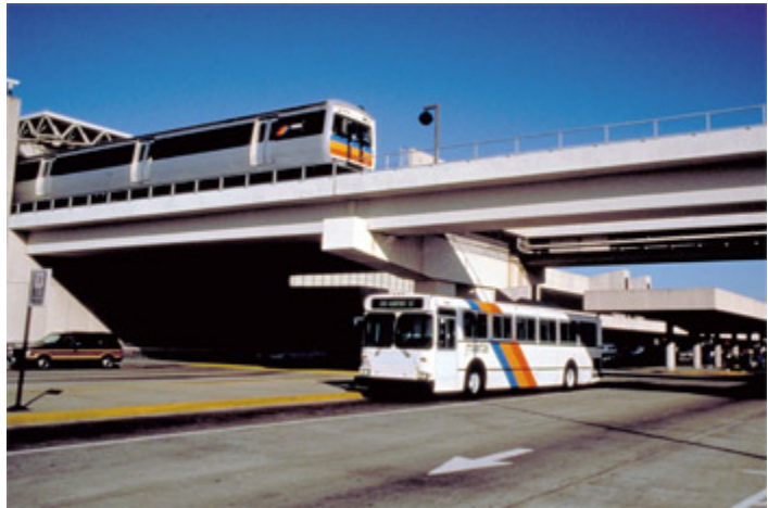
Photo courtesy of Metropolitan Atlanta Rapid Transit Authority
