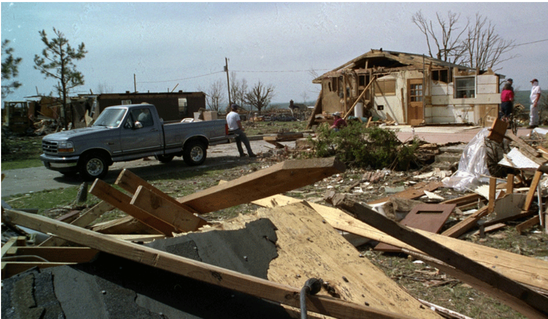
Another scene of residential destruction from August 24, 1992, in Dade County, Florida. Photo by Bob Epstein and courtesy of the Federal Emergency Management Agency
