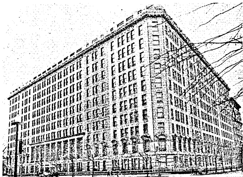
Veterans Administration Building, Washington, D. C.
